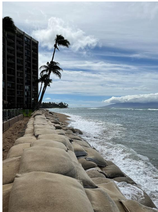
Sandbags and other geotextile materials may act as a temporary emergency measure to protect backshore infrastructure until a better solution can be implemented, but their presence often exacerbates erosion on sandy beaches. (Photo credit: SSFM)
