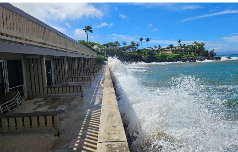
Retreat may be considered for areas experiencing severe coastal hazards, such as Kahana Sunset Building F in West Maui, November 2023 (Photo Credit: SSFM)
