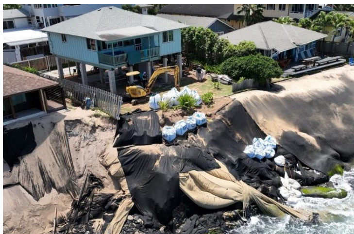
Geotextile burritos, sandbags and skirts have exacerbated beach loss in the study area. This home was moved back and elevated in response to the erosion threat. (Photo credit: DLNR)
