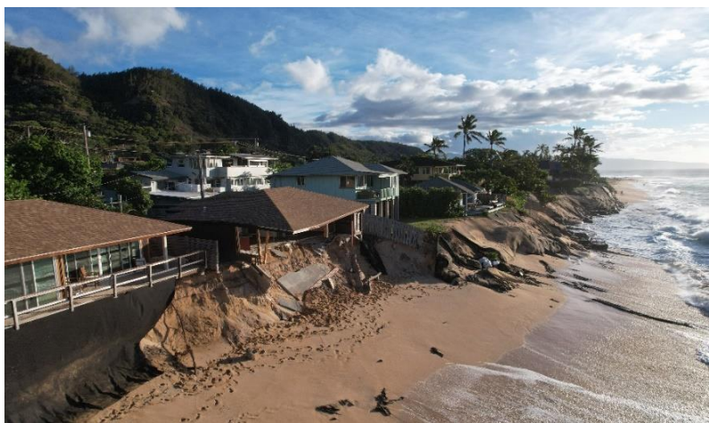
A house collapses onto the beach near Sunset Beach on the North Shore of O'ahu, September 2024 (Photo Credit: Rob Walker/Integral Consulting)
