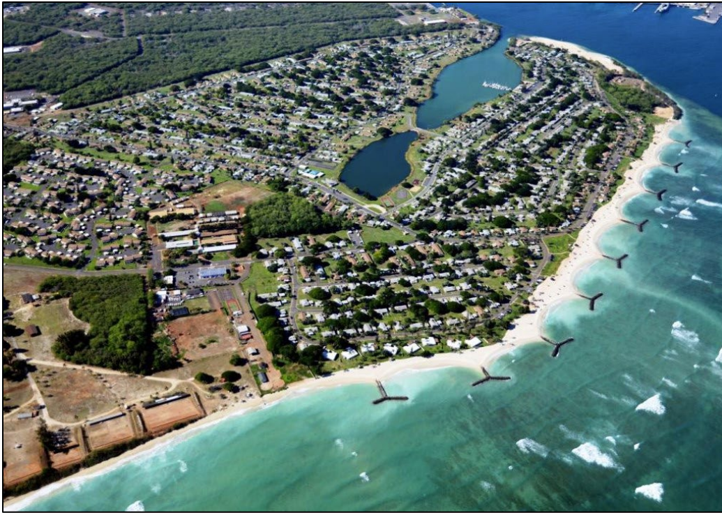
Figure A3-8. Beach nourishment with stabilizing groins at Iroquois Point, O'ahu
