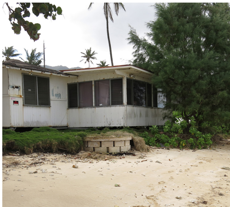
Cesspool in Punalu‘u, O‘ahu exposed by chronic coastal erosion. Source: DNLR, Office of Conservation and Coastal Lands photo archive
