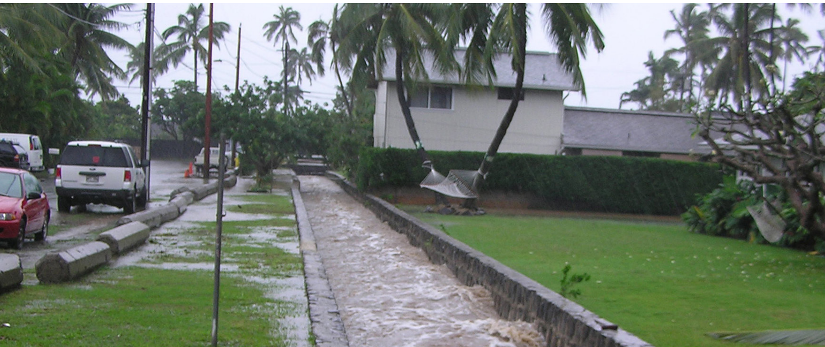
Lanipo drainage in Lanikai, O'ahu. Source: The Nature Conservancy, Andrew Hood
