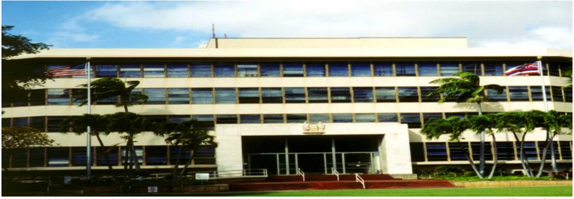
The Queen Liliuokalani Building on 1390 Miller Street in downtown Honolulu houses the administrative offices of the Department of Human Services.
