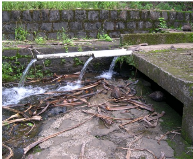
Bypass pipes at Haiku Ditch, Honopou Stream
