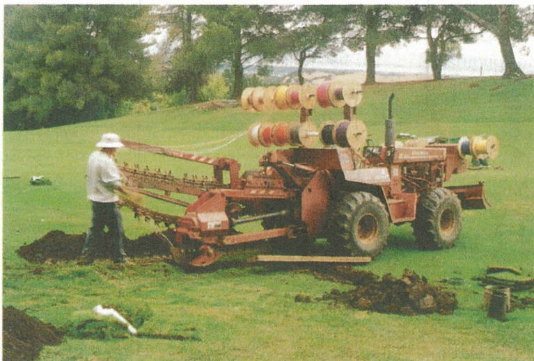
Figure 9.26. A pipe-pulling machine positioned at the pipe entry point (top) and in operation (bottom).
