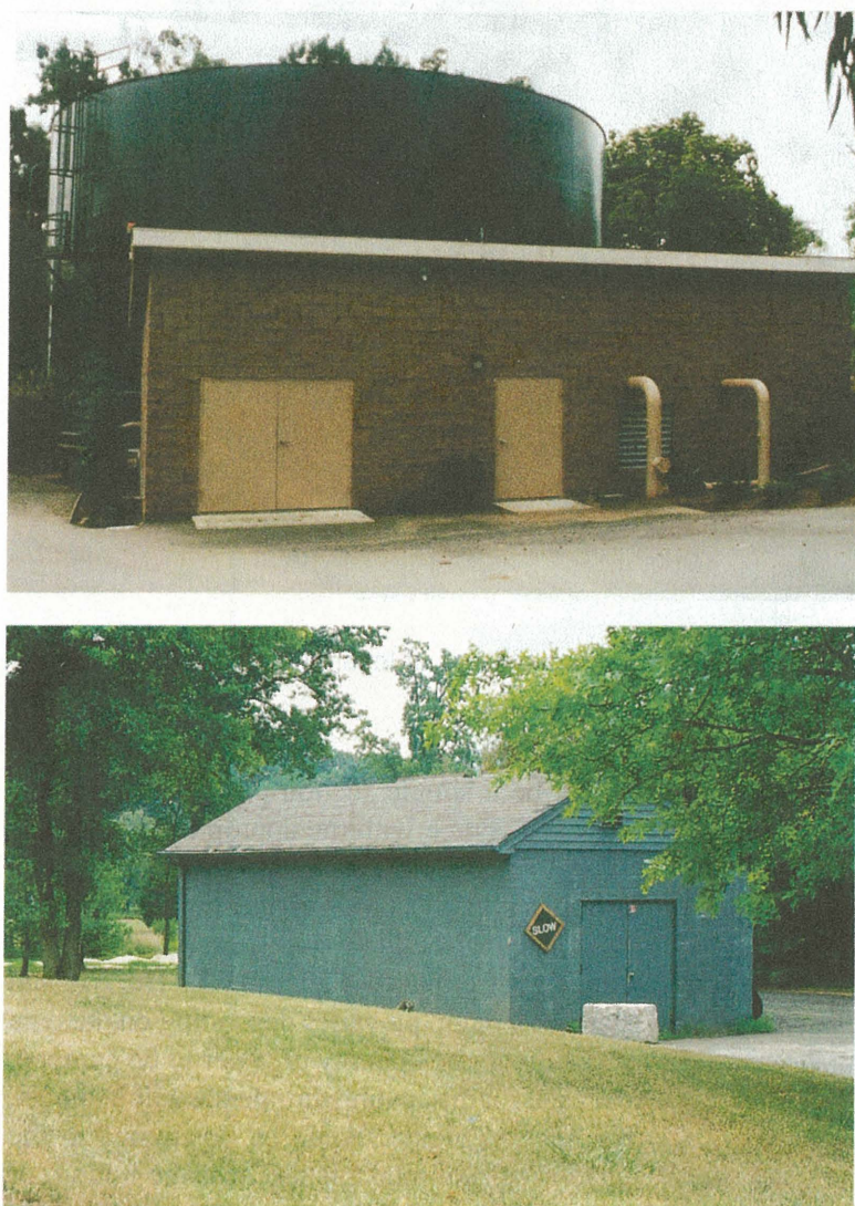
Figure 9.22. Two types of permanently constructed pump houses. (top—Courtesy of P.M. Hathaway.)
