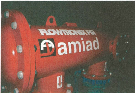
Figure 9.4. A mechanical strainer used to clean a raw water supply containing debris.
