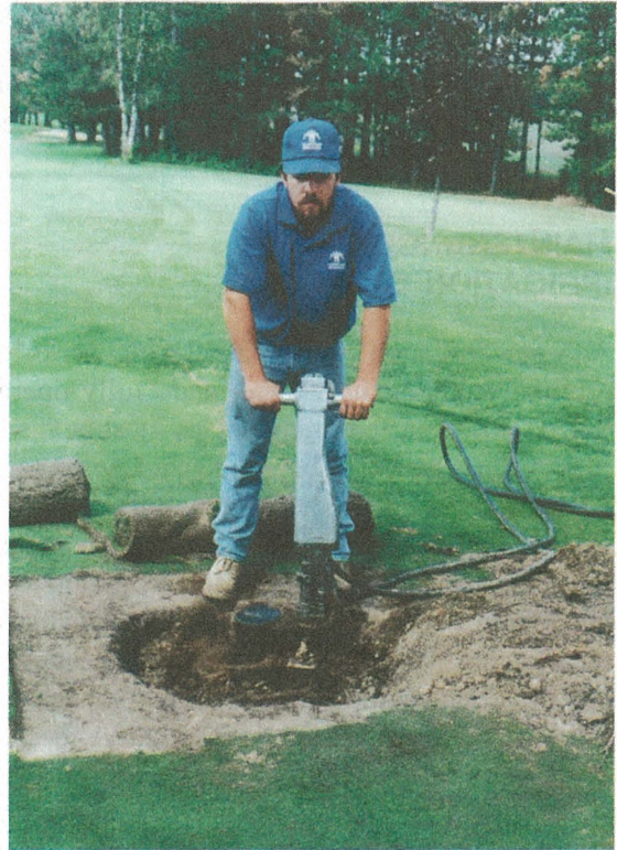
Figure 9.29. A powered tamp being used to firm the soil around a sprinkler head. (Courtesy of The Toro Company.)
