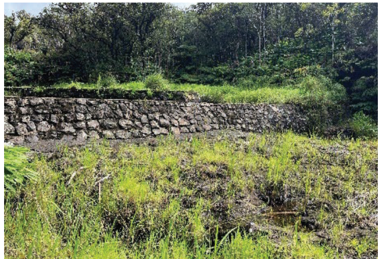
Upstream view of Hawai'i DWS dam
