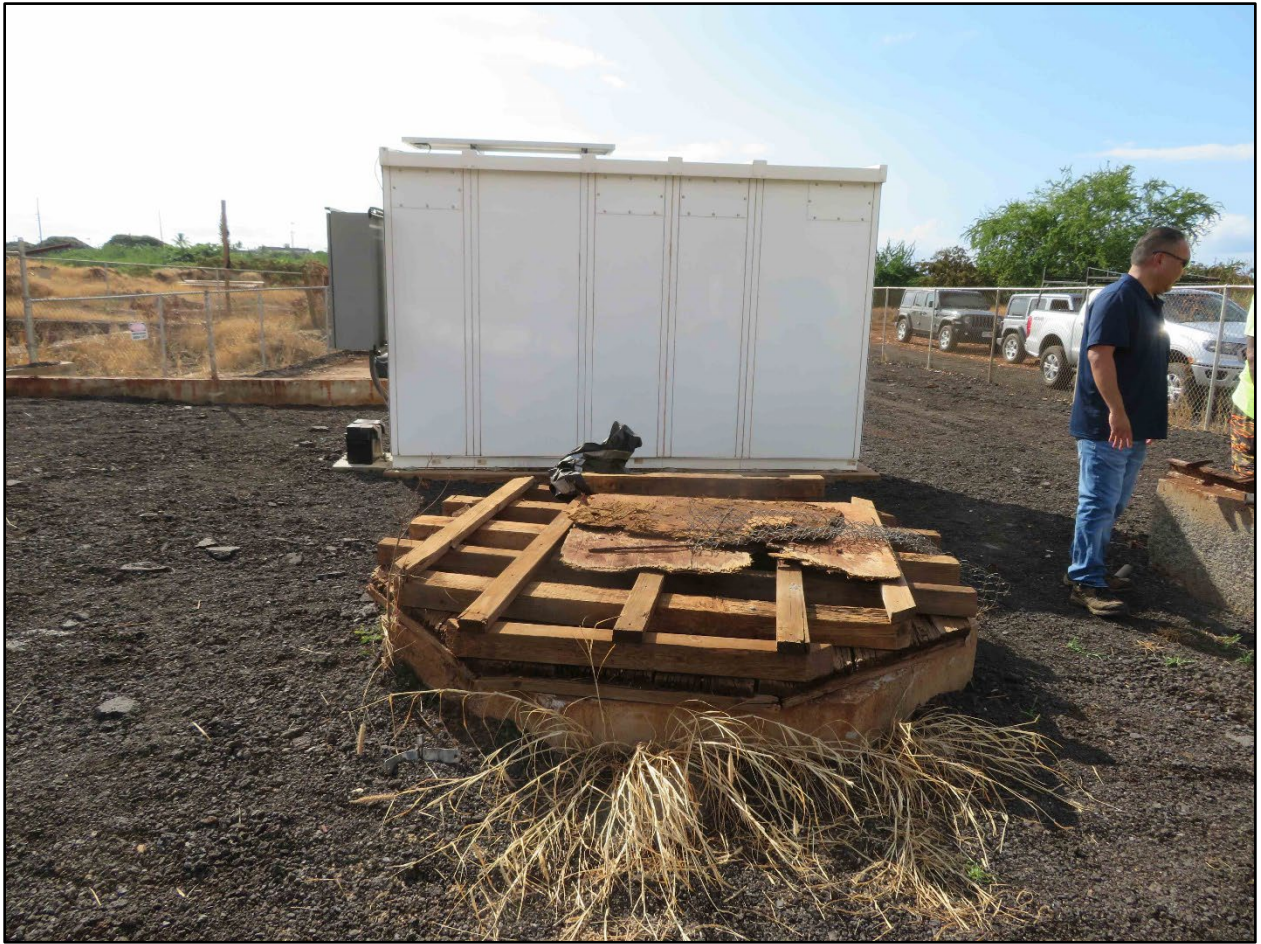
Shaft located between the two Pump Houses, opened to surface exposure, Looking Northwest
