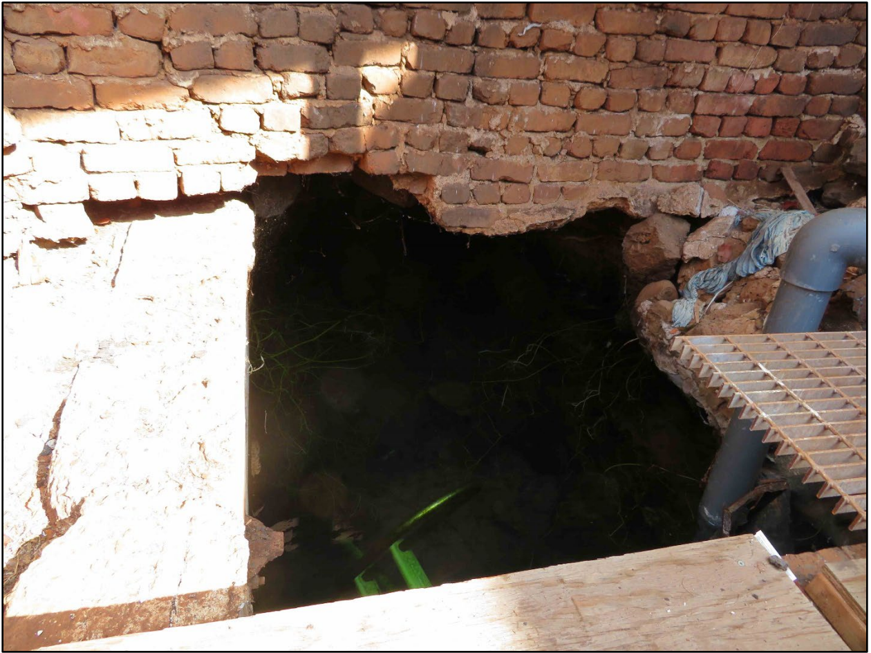
Tunnel at east side of Shaft Pump House looking Directly Northeast
