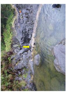
View downstream of diversion pool site gh063r-040208. Black 6'PVC pipe (yellow arrow) in the middle is carrying water downstream. Upper reach Pi'ina'au Stream, Maui, Hawai'i.
