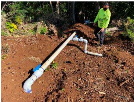
C) Newly installed lateral 4-inch line from Waikapū Properties’ line continues to South Waikapū Kuleana ‘Auwai.
