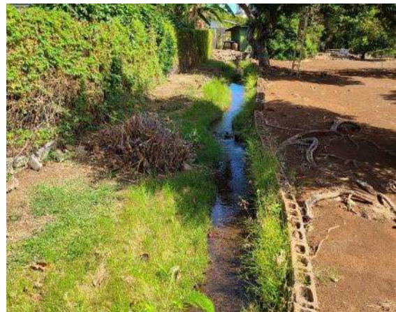
B) Water flows underground from Imua Family Services and drops into an open ditch on the Koeli LLC property.
