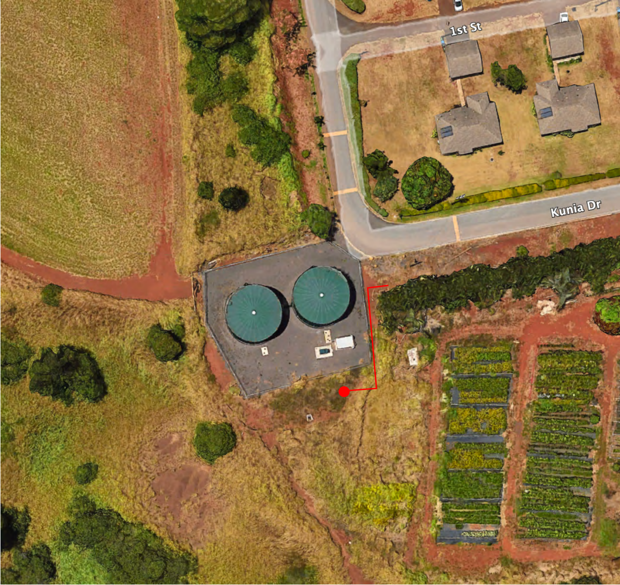
Well site and piping to connect to existing filter station
