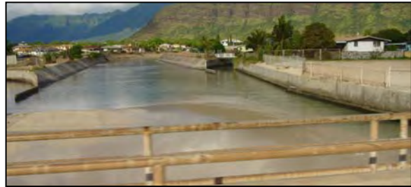
Flood control drainage canal.
