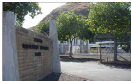
Wai’anae Wastewater Treatment Plant.
