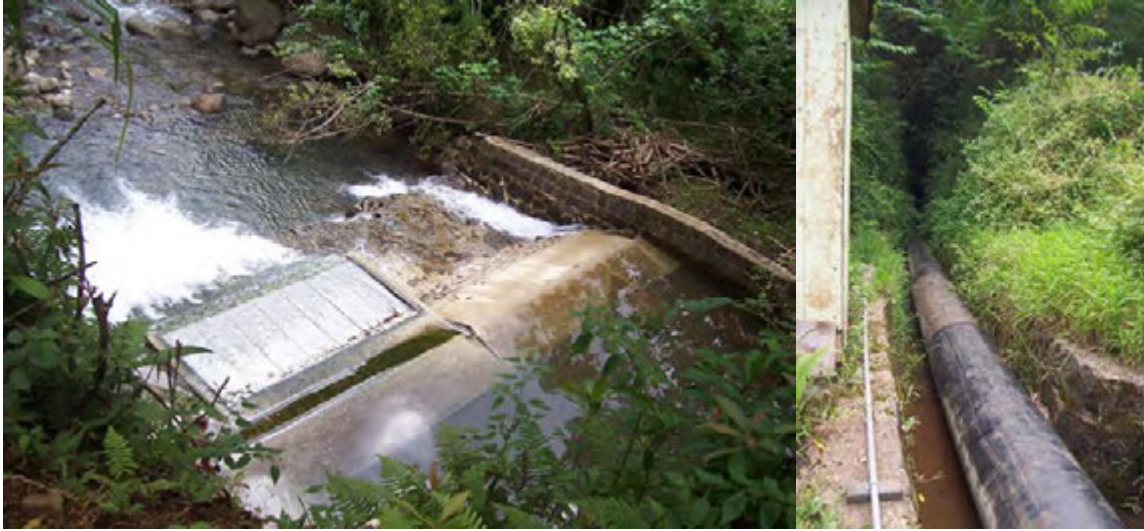
Figure 1.6 Punalu'u Stream Diversion and Piped Ditch
