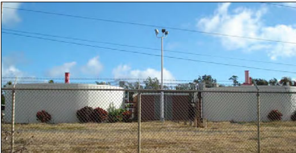
Waimānalo WWTP facility
