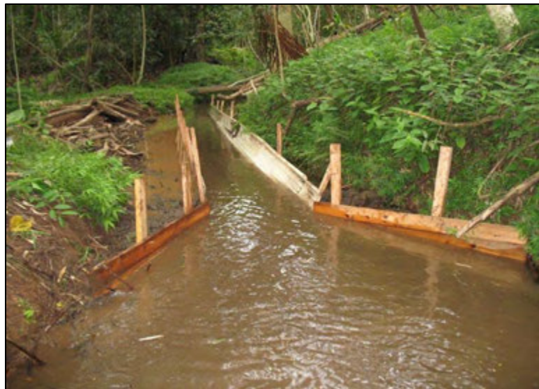
Temporary upgrades of the Waimānalo Irrigation System
