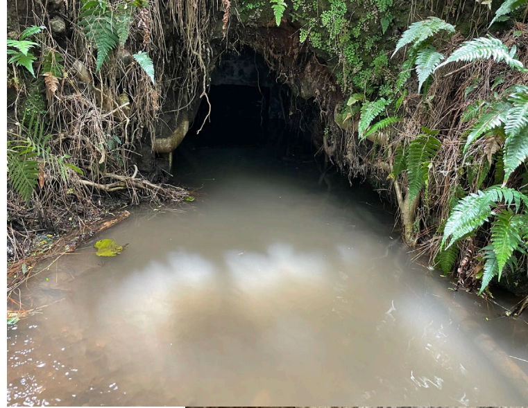
Murphy Tunnel (well 8-7145-002)
