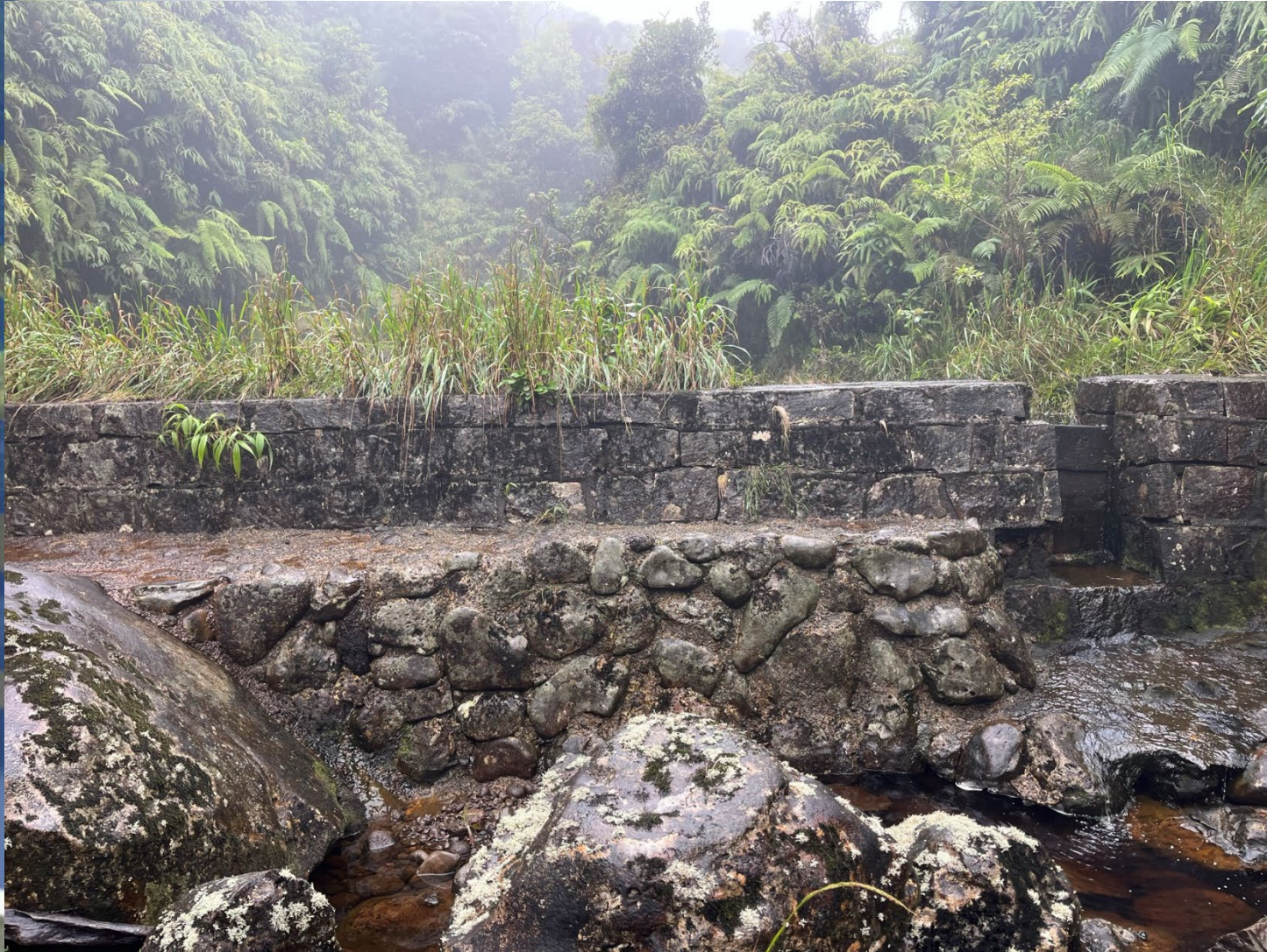
Diversion dam on Kawainui Stream
