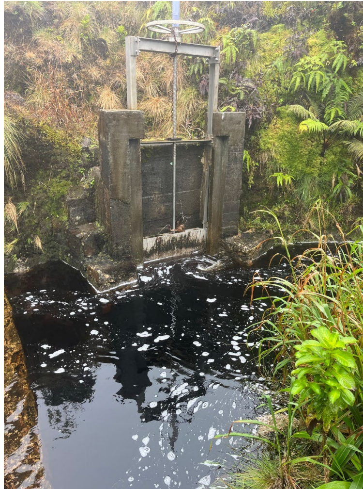
Diversion intake on Kawaiki Stream
