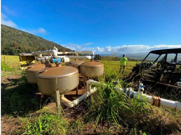
9) Sand filters located on the main 8-inch line from Reservoir 1.
