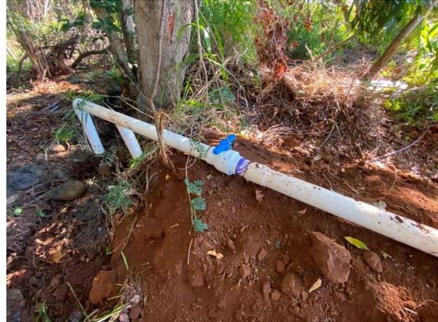
16) End of lateral 4-inch line at drop point to South Waikapū Kuleana ‘Auwai. Little flow was noted in the ‘auwai. CLA (pressure-reducing) valve will be installed before the last ball (control) valve to the ‘auwai.
