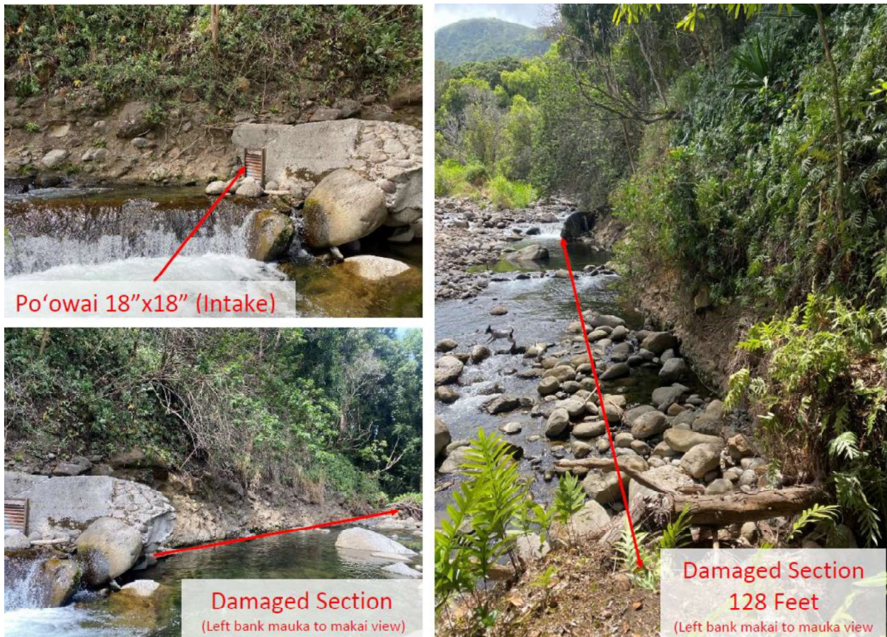
1D. Collage of damaged 'auwai section details. A) Image at upper left is looking towards the left bank with the intact concrete headwall or po'owai; B) Image at lower left is looking towards the left bank and downstream showing the damaged section of the 'auwai; C) Image at right is the damaged 'auwai section on the left bank, looking upstream.
