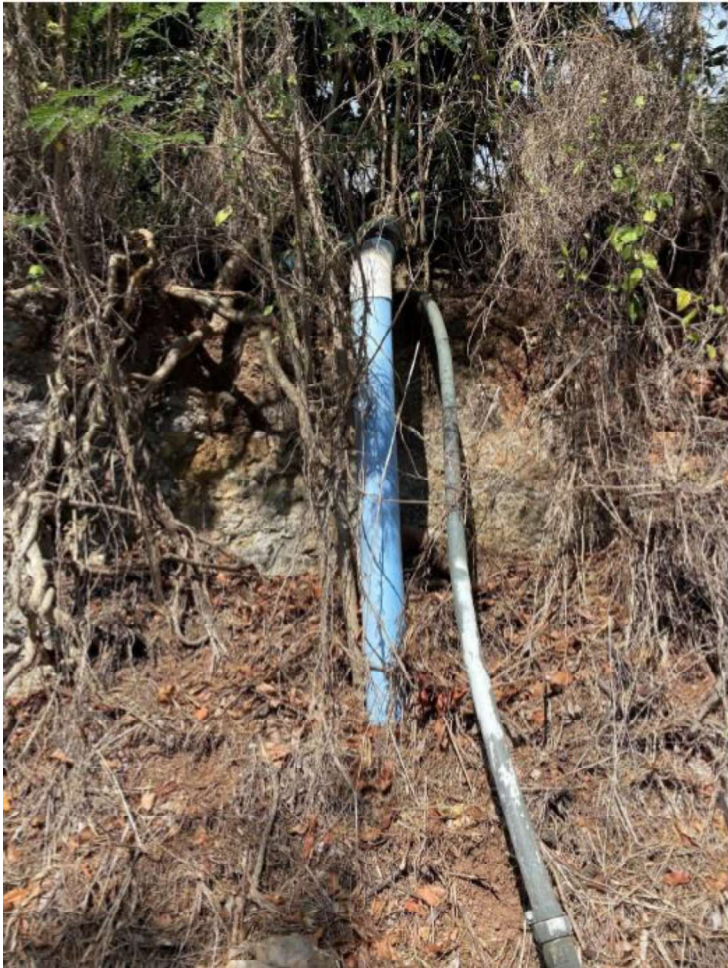
1E. The six (6) inch pipe (blue) under the Kahekili Highway provides water to the makai side of the highway and the last permittee.
