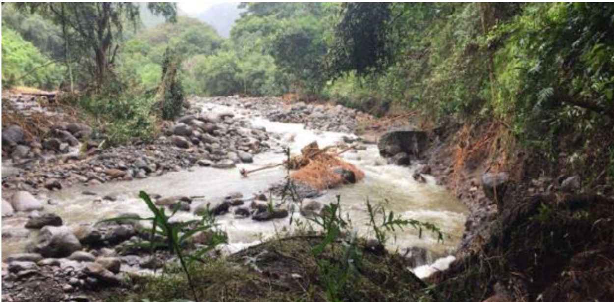
1B. Waihe'e River, looking upstream, following a flood event and the loss of the 'Auwai intake in 2018. Note the concrete intake structure is visible in the center right, along the left bank of the river.
