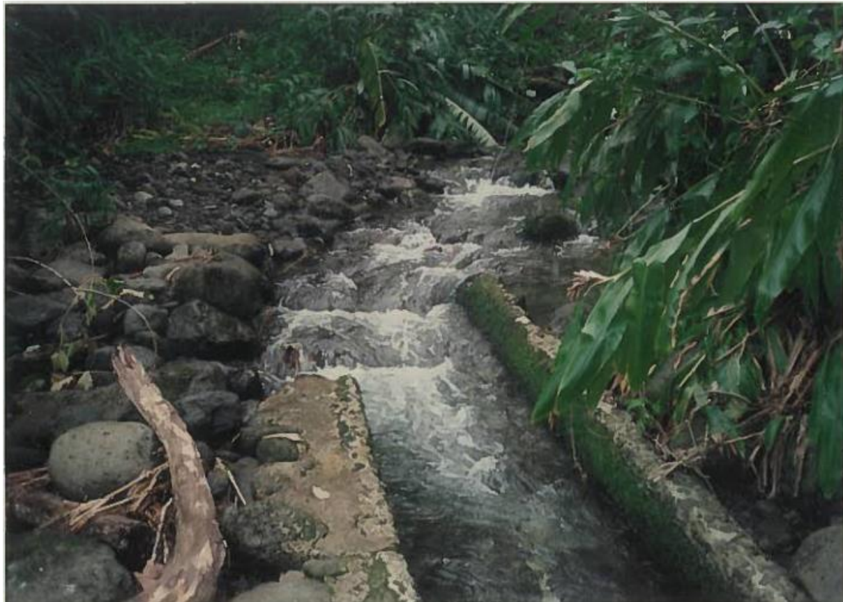
2C. North Waiehu Stream, looking upstream, flowing into the ditch. Photo taken by Commission staff, March 1989.
