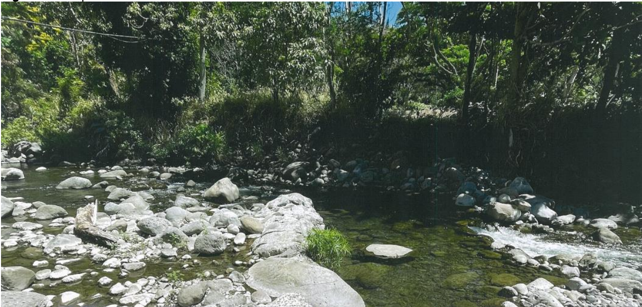
3A. Wailuku River looking north and upstream, concrete apron partially across the stream at center.
