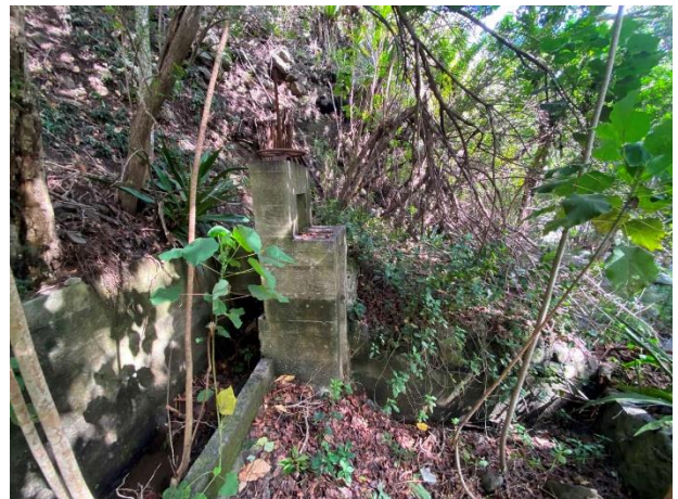
2D. Water is returned to Waikapū Stream via this sluice gate on the left bank approximately 200 ft. away from the intake.
