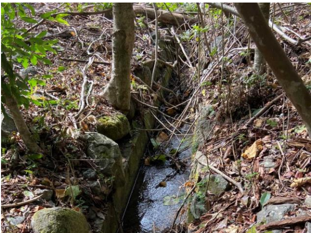
2C. Everett Ditch continues to receive a small amount of water from the intake on Waikapū Stream.
