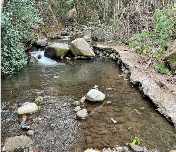
2A. Waikapū Stream looking upstream. Concrete diversion structure on the right.
