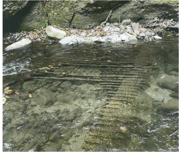
2B. Waikapū Stream from the left bank looking south. The remnant intake grate is filled with rocks and debris.
