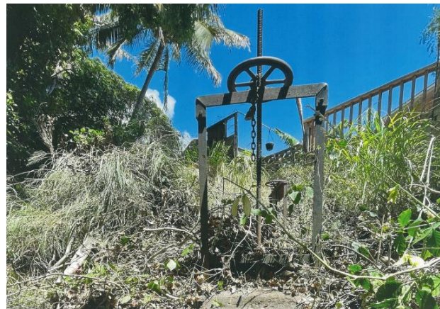
3B. Closed gate valve located on the left bank of Waikapū Stream.
