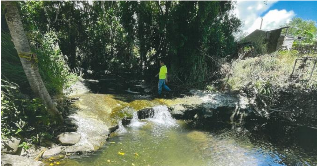
3C. Waikapū Stream looking upstream. An overhanging concrete lip is located just below the diversion intake with closed gate valve on the left bank of the stream (right side of photo).
