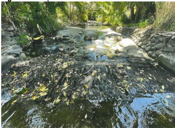
3A. Waikapū Stream looking downstream with diversion intake grate in the foreground.
