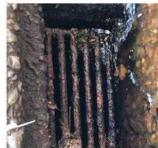
PICTURE OF EXISTING INTAKE BOX OPENING AND GRATE
