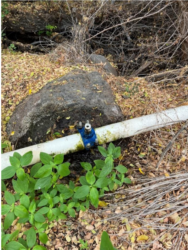
c) Leakage from Olowalu Cultural Reserve pipeline below meter
