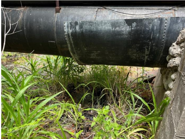
a) Water leakage from Lower Olowalu Ditch flume
