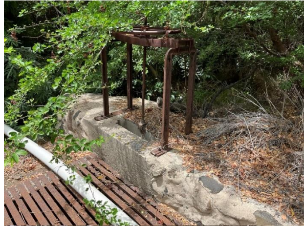
b) water leakage from Lower Olowalu Ditch sluice gate.
