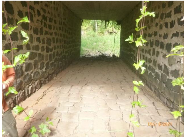
Stream channel upstream of the culvert, looking downstream.
