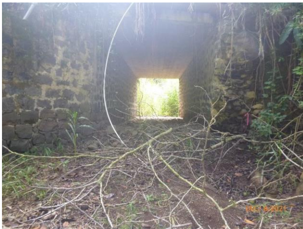
Stream channel at the project area, looking upstream.
