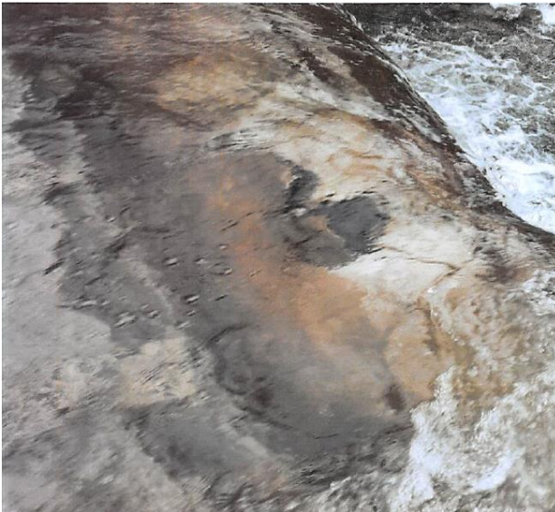
C) Close-up of the hole in the Waihee Ditch siphon.
