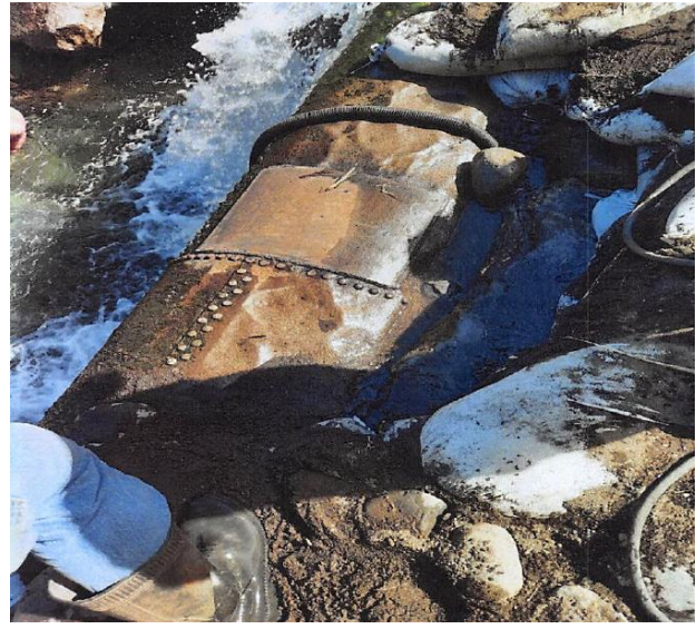
D) 24-inch x 20-inch steel plate welded over the hole in the siphon
