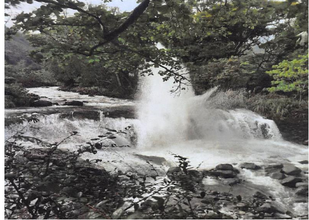
B) View upstream of geyser at broken Waihee Ditch siphon, from right bank, December 5, 2021.
