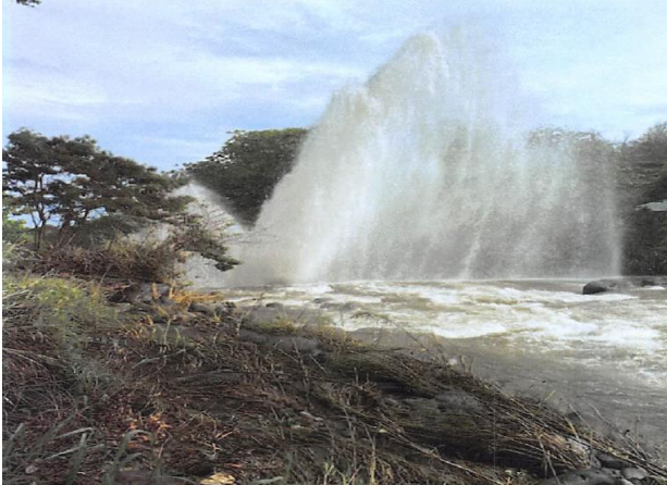
A) View downstream of geyser at broken Waihee Ditch siphon, from left bank, December 5, 2021.
