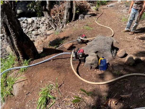
Site E: 1-inch hoses attached to two 32 gpm pumps on TMK (2) 4-5-016:888, right bank of Kahoma Stream. (Note: Applicant is only applying to use one 32 gpm pump.)
