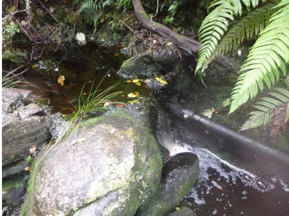
Close-up view of diversion dam and diversion intake pipe on left bank of stream.
