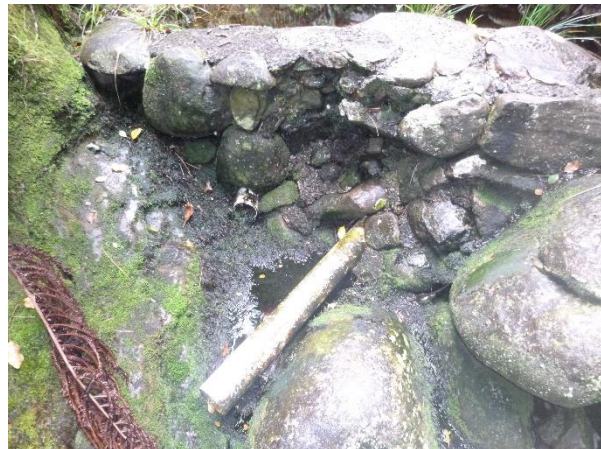
Close-up view of diversion dam and remnant pipe.
