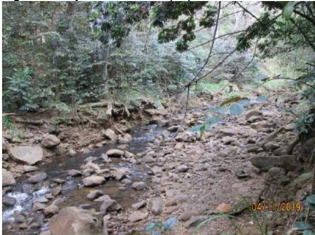
Looking upstream at approximate location of DL No. 2 outlet and stream stabilization.
