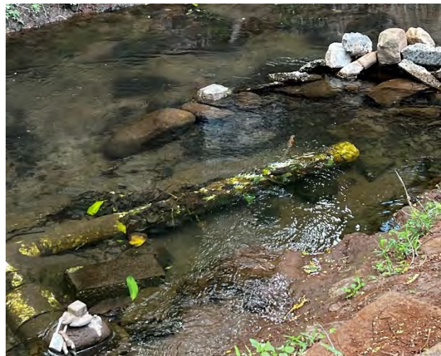
Close up of diversion located in the Waihe'e Ditch.
