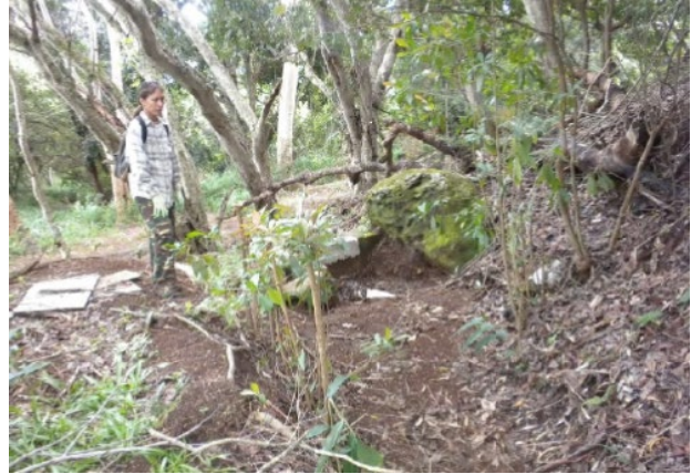
Cement basin connecting to "white pipe". Shared source with Nakama.
