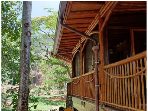
Rain catchment system.
