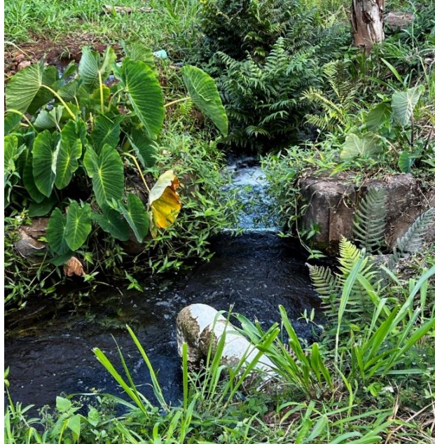
8-inch kuleana pipe at start of north and south side 'auwai. Looking makai toward Malaihi Road.
