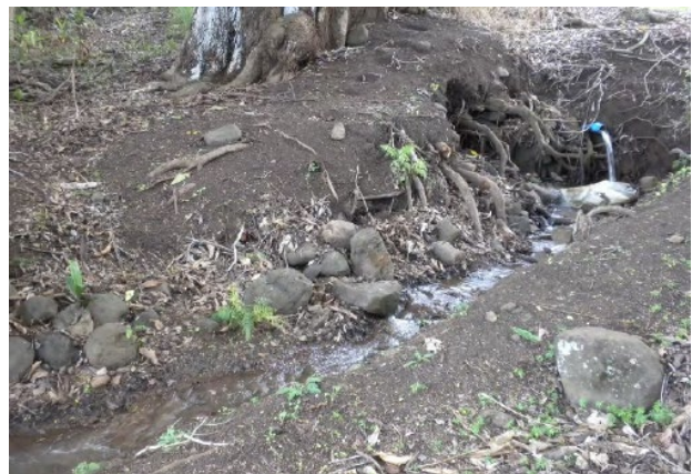
"White pipe" exiting into Hoopii property.
