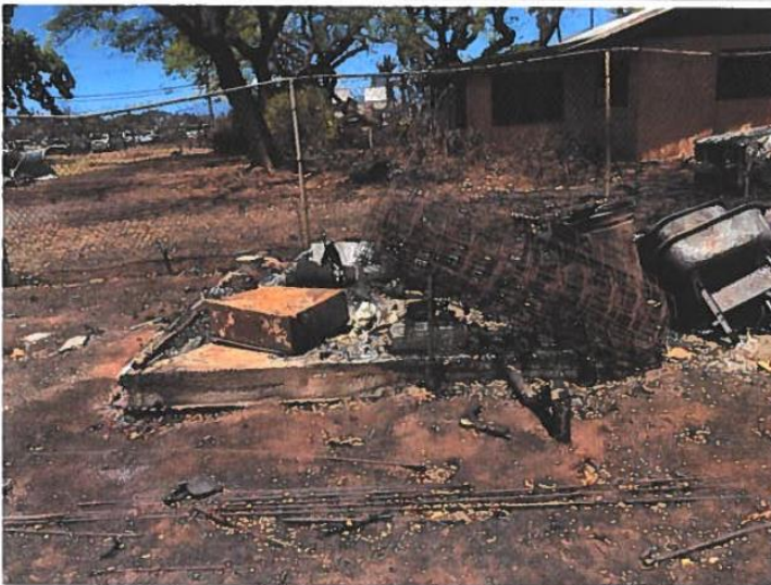
11 Well 6-5240-005 (Methodist Church)
