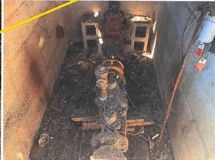
2 Well 6-5240-001 Under metal covers
