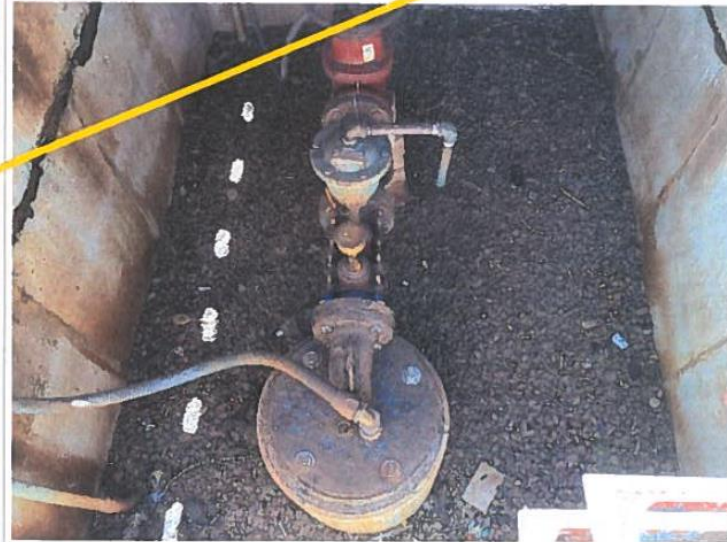
14 Well 6-5240-007 , Under metal covers
