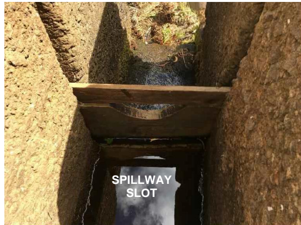
Overhead close-up view of the spillway slot in the diversion dam (KIUC, 2020).
