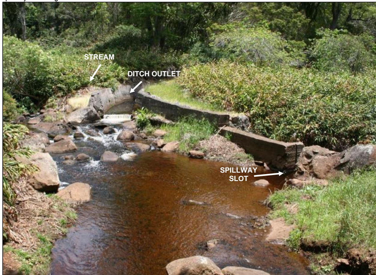
Figure 7. Kōke'e Stream from right bank, looking towards Kōke'e Ditch dropping water into Kōke'e Stream, with spillway slot at right.
