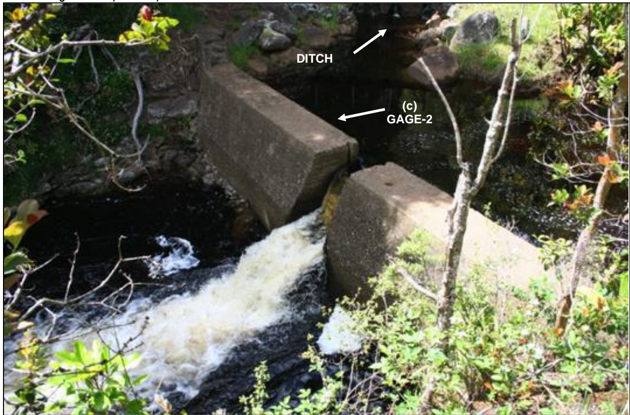
Figure 5. Kauaikinana diversion showing the stream entering from the right, flowing through the stoplog slot and the ditch exiting to the top of the photo.
