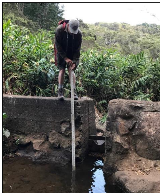
Figure 9. Location of BPT and Staff Gage at spillway slot on Kōke'e Stream diversion dam.
