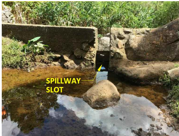
Downstream view of the spillway slot in the diversion dam (KIUC, 2020).
