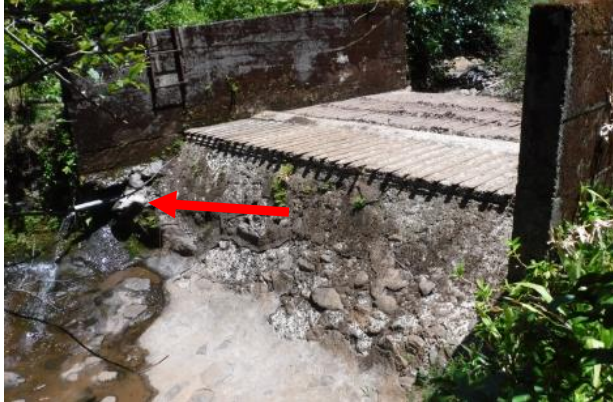
Upstream view of bypass channel with bypass pipe at right bank (Sierra Club, 2020).
