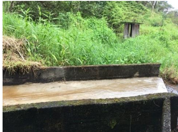
Diversion intake structure after sealing (EMI, 2020).
