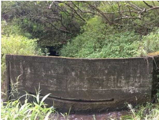
Diversion structure before sealing (EMI, 2020).
