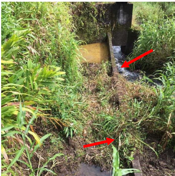
Diversion structure after sealing (EMI, 2020).
