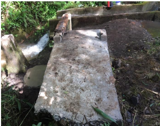
Diversion structure after sealing (EMI, 2020).
