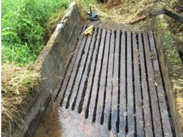
Diversion intake structure before sealing (EMI, 2020).
