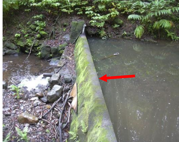
Diversion dam and collection pond, with bypass pipe, taken from left bank (CWRM, 2009).
