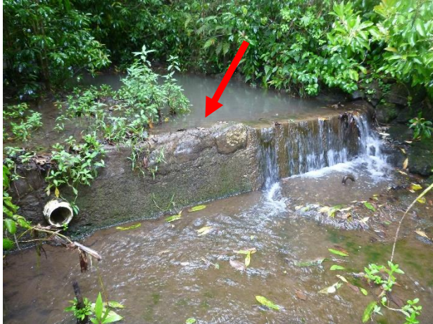
Upstream view of diversion dam and intake on left bank (CWRM, 2016).
