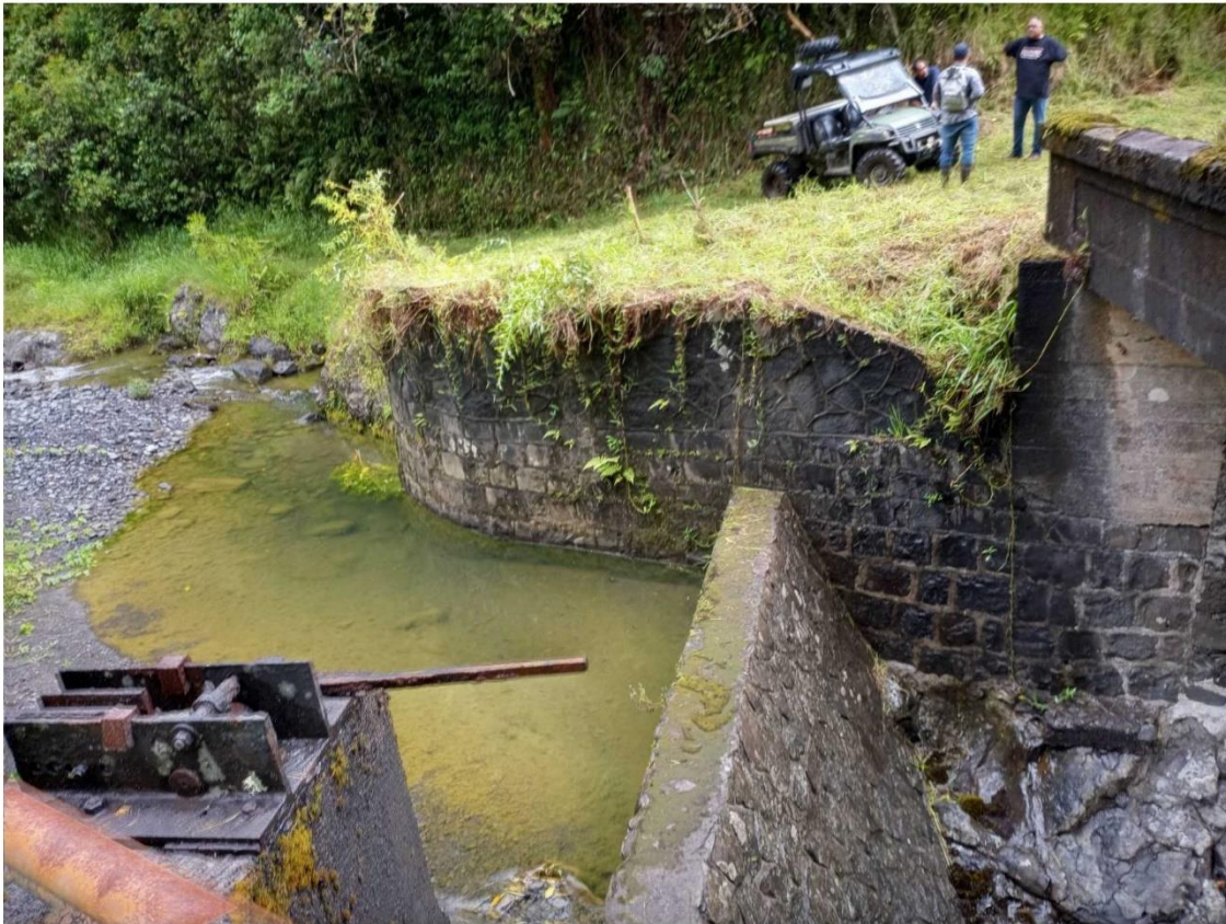
Photo 3. Rockwall supported embankment on the west side of the bridge and dike.
