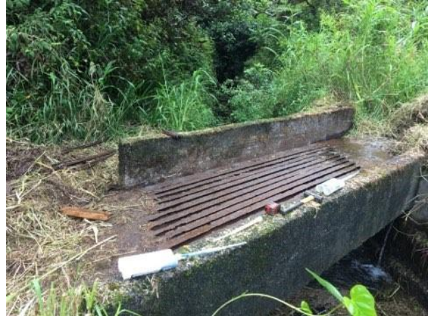
Diversion intake structure before sealing (EMI, 2020).
