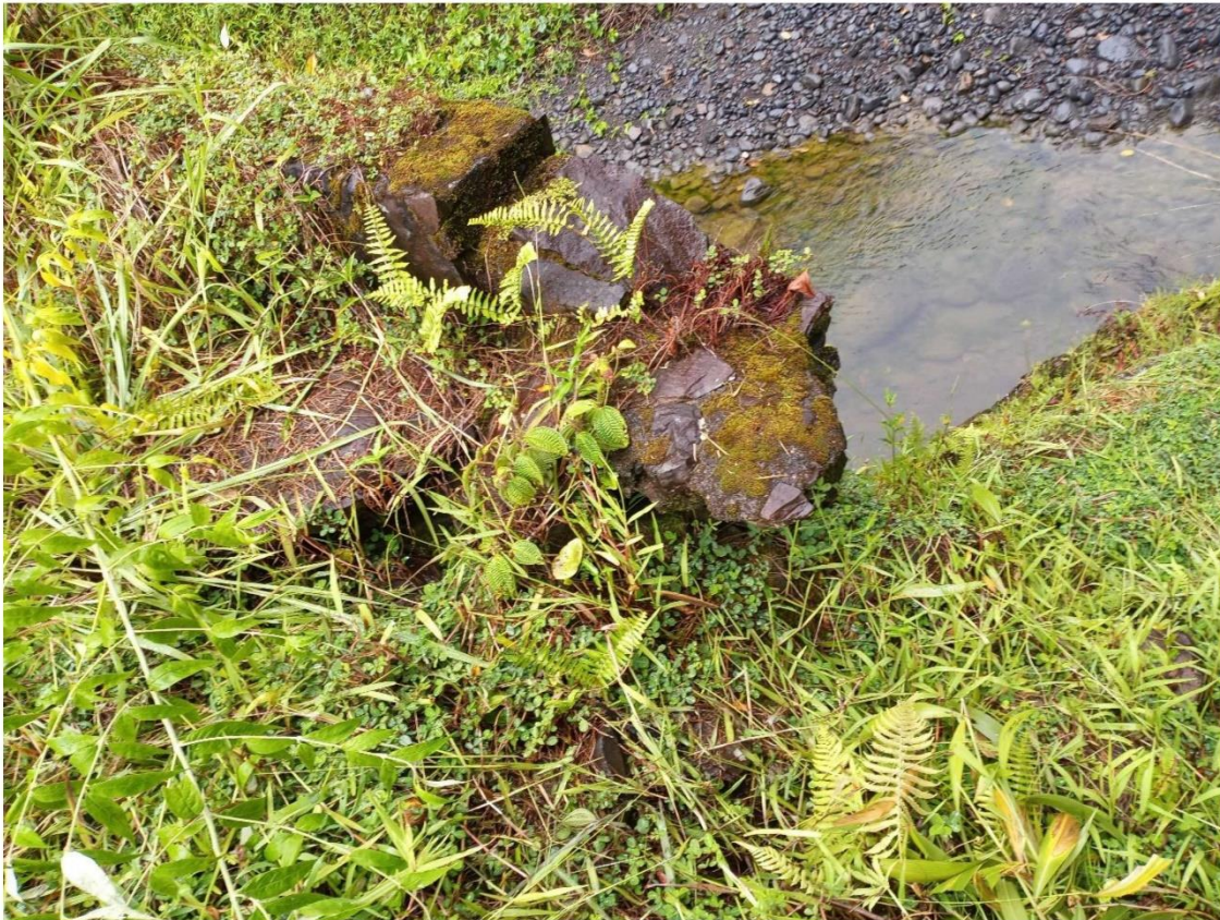
Photo 4. View of the crumbling rockwall supported embankment at its west side.
