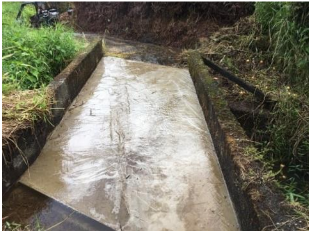
Diversion intake structure after sealing (EMI, 2020).
