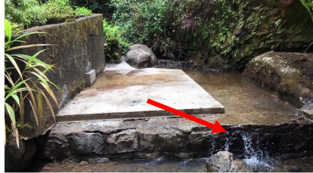
Diversion structure after sealing (EMI, 2020).
