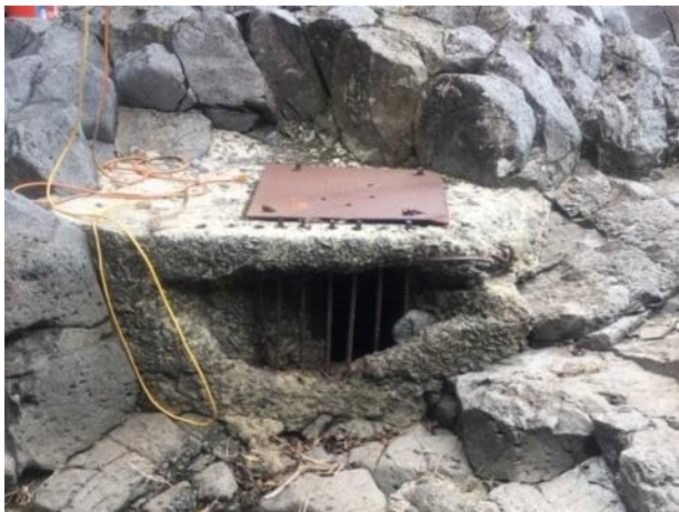
Diversion structure before sealing (EMI, 2020).
