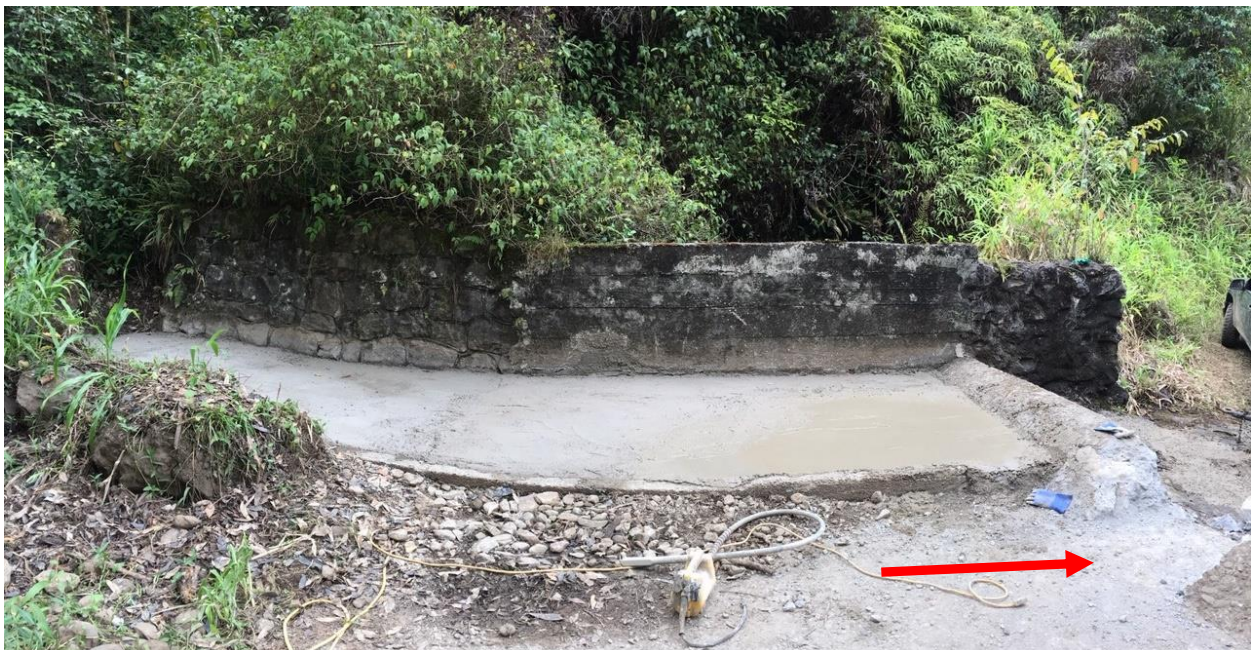
Diversion structure after sealing (EMI, 2020).
