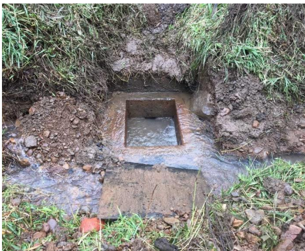
Diversion structure before sealing (EMI, 2020).
