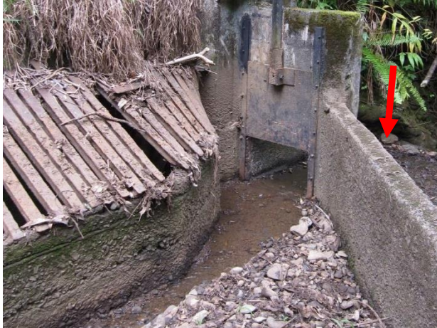
Diversion intake structure (CWRM, 2009).
