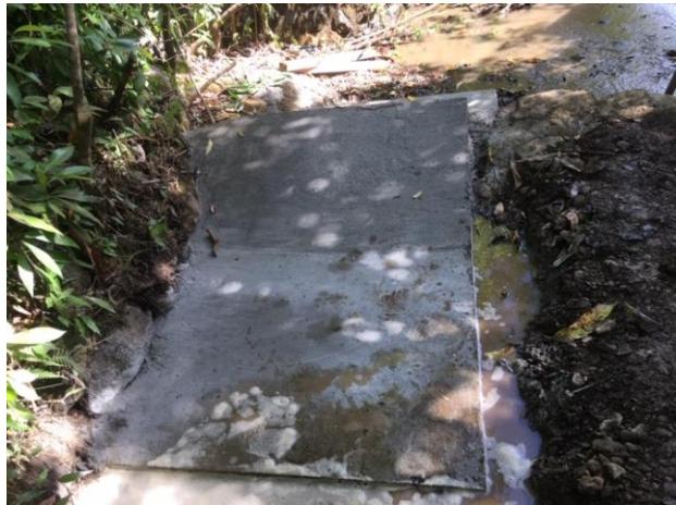
Diversion structure after sealing (EMI, 2020).
