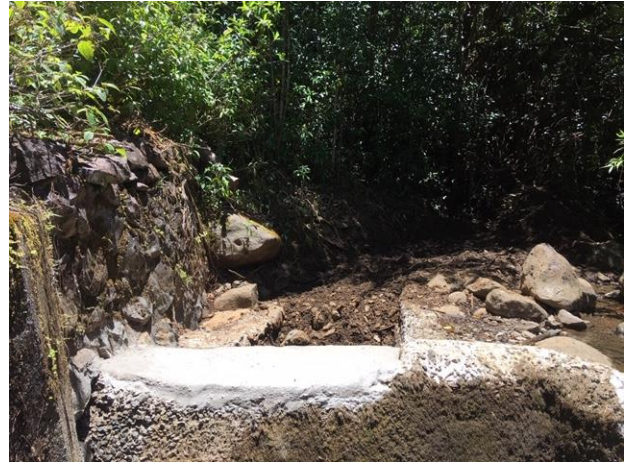
Diversion structure after sealing (EMI, 2020).
