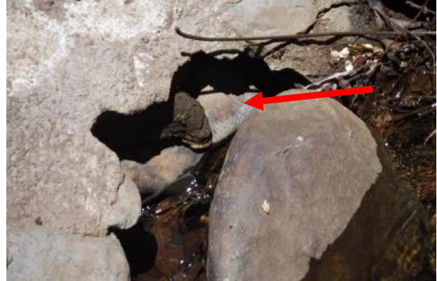
Close-up view of leak into Lowrie Ditch on upstream end of bypass channel (Sierra Club, 2020).
