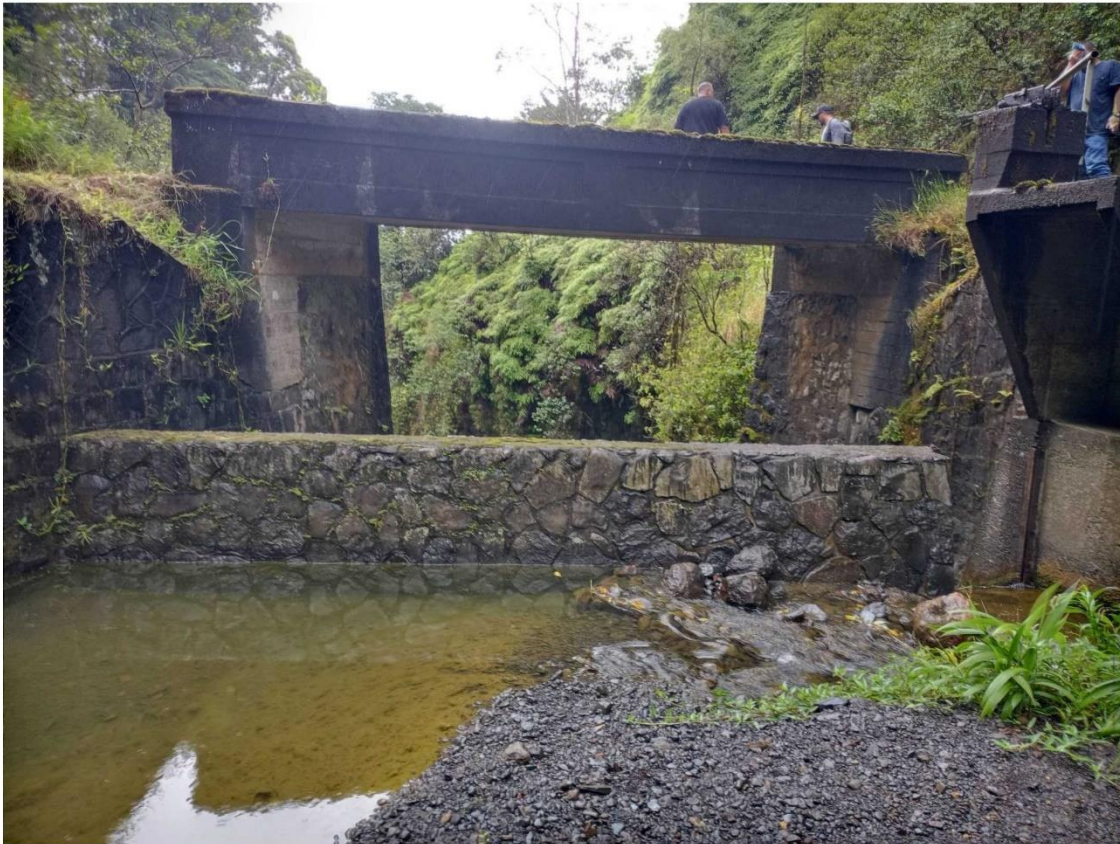
Photo 2. View of the impermeable dike on the river bed.
