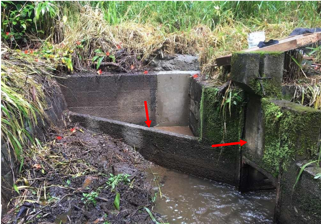
Diversion structure after sealing (EMI, 2020).
