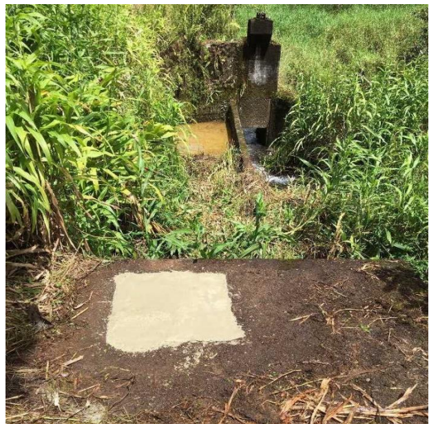
Diversion structure after sealing (EMI, 2020).
