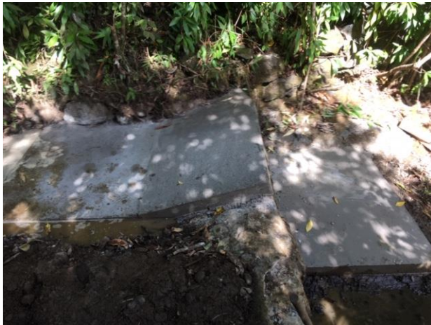
Diversion structure after sealing (EMI, 2020).
