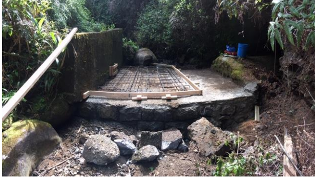
Diversion structure before sealing (EMI, 2020).
