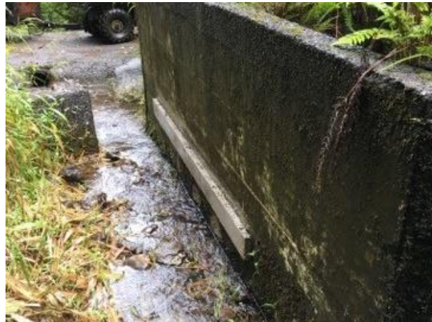
Diversion structure after sealing (EMI, 2020).
