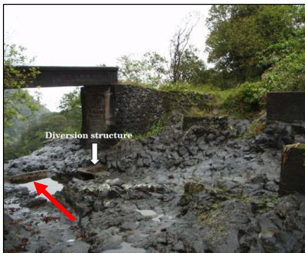
Diversion intake structure on right bank (DAR, 2008).
