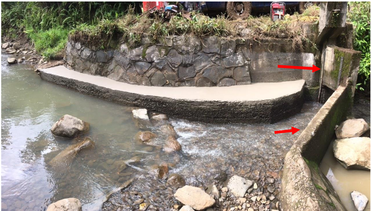
Diversion intake structure after sealing (EMI, 2020).
