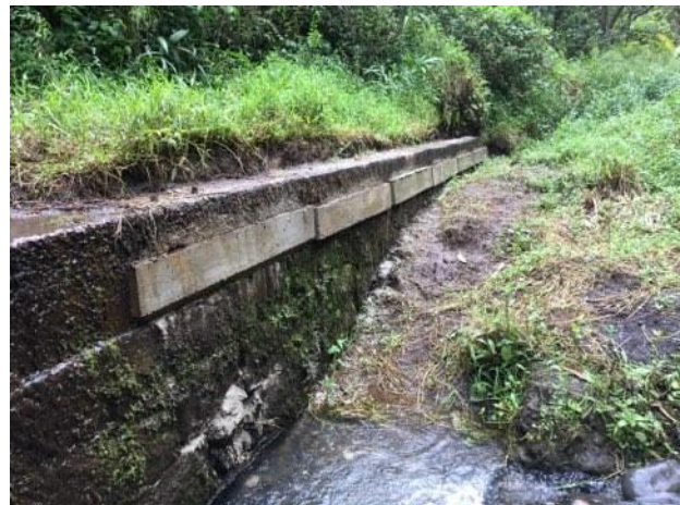
Diversion structure before sealing (EMI, 2020).
