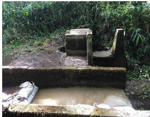
Diversion structure after sealing (EMI, 2020).
