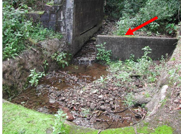
Upstream view with water flowing downstream after control gate removed (CWRM, 2008).
