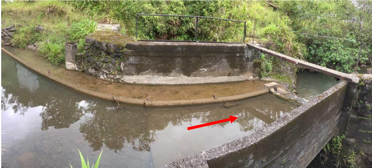
Diversion structure after sealing (EMI, 2020).
