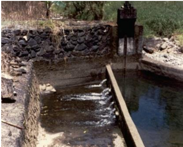
Downstream view of stream ponding behind the sluice gate, where it then passes through holes in the wall and drops into the ditch below the intake (EMI, 1989).
