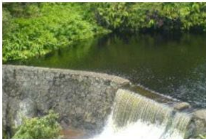
Hawai'i Department of Water Supply diversion intake at Kohākōhau Stream.
