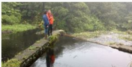
Hawai'i Department of Water Supply diversion intake (Marine Dam) on Waikoloa Stream.
