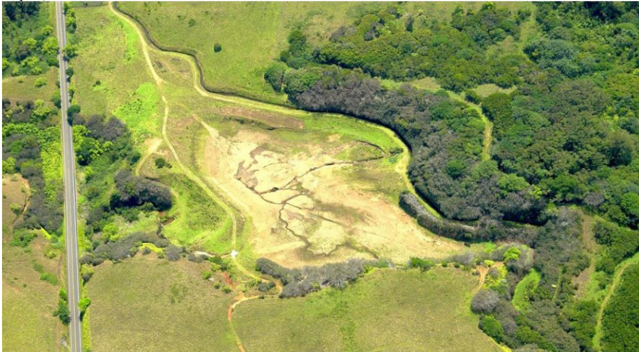
Figure 2: Site Photo, Kapala‘alaea Dam, looking east. Source: Hawaii DLNR Dam Inventory System; image date May 10, 2007.
