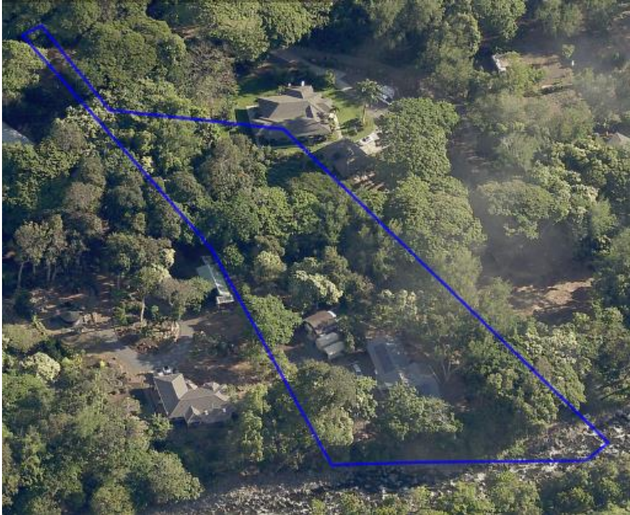
Figure 2: Subject location on Wailuku River, Maui. Photo date 6.28.2022. From the County of Maui website.
