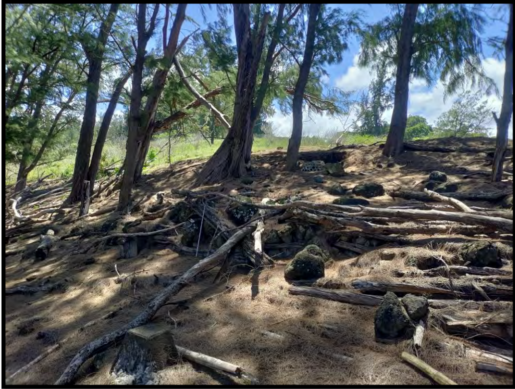
Figure 31. Site 31350, downslope retaining wall of angular stones (pier block in foreground, mortar block with bottles in background; view to south).
