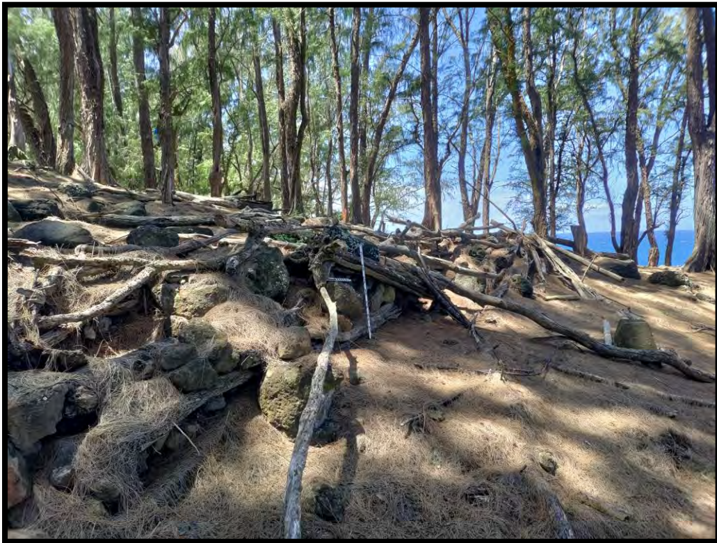
Figure 30. Site 31350, downslope retaining wall of angular basalt stones (pier block on right; view to west).
