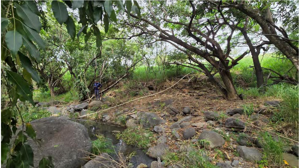
Figure 10.b. Unidentified Stream Diversion #1, approximately 780 feet downstream from Haleahi Rd. and Kaupuni Stream crossing.
