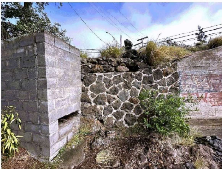
13. Downstream of Waiaka Bridge at Embankment. Multiple foundations in proximity. Note exposed reinforcing steel at top of concrete block wall.
