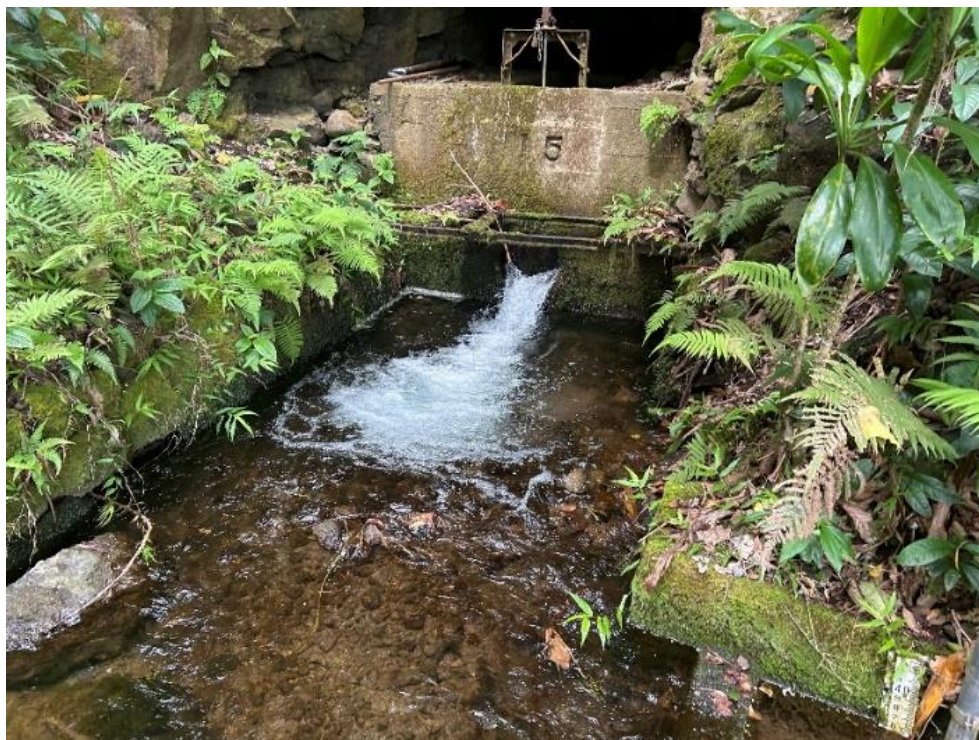
Figure 3a. Picture of Adit 15 (Taro Gate) return flow from Honokōhau Ditch to Honokōhau Stream.
