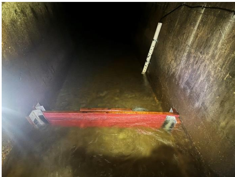
Figure 5b. Downstream view of stoplog board installed downstream of Adit 15 in Honokōhau Ditch to increase the returned flow through Adit 15 on April 15, 2025
