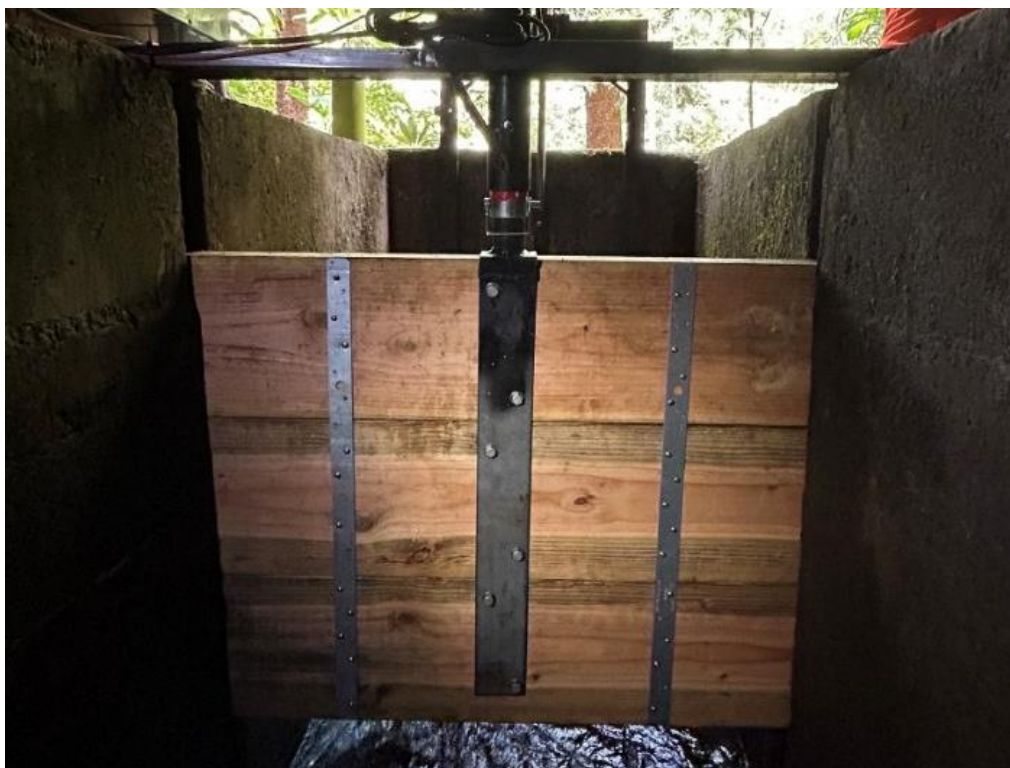
Figure 3b. Remotely operable board installed downstream of Adit 15 in Honokōhau Ditch to increase returned flow, June 14, 2025.
