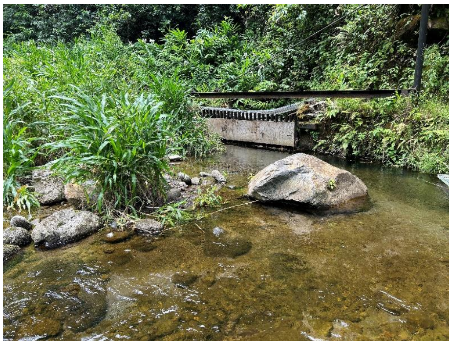
Figure 6b. Temporary high-flow restrictor at Aotaki Weir intake.
