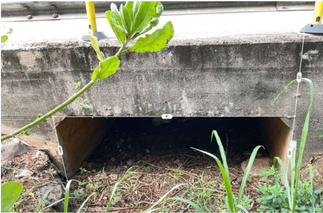
Figure 3-12. Existing Box Culvert#3 on Kamehameha Highway (Site Survey Photo)
