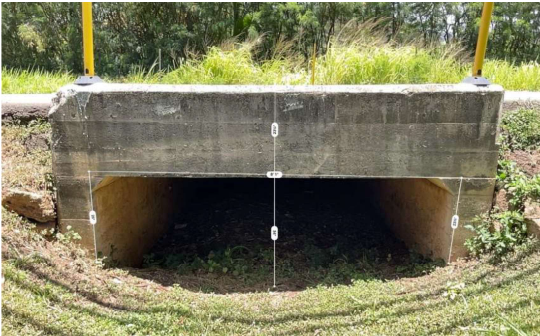
Figure 3-10. Existing Box Culvert#1 on Kamehameha Highway (Site Survey Photo)
