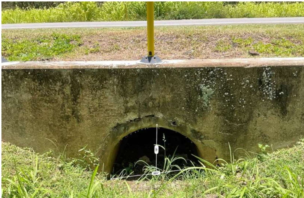
Figure 3-13. Existing Pipe Culvert on Kamehameha Highway (Site Survey Photo)
