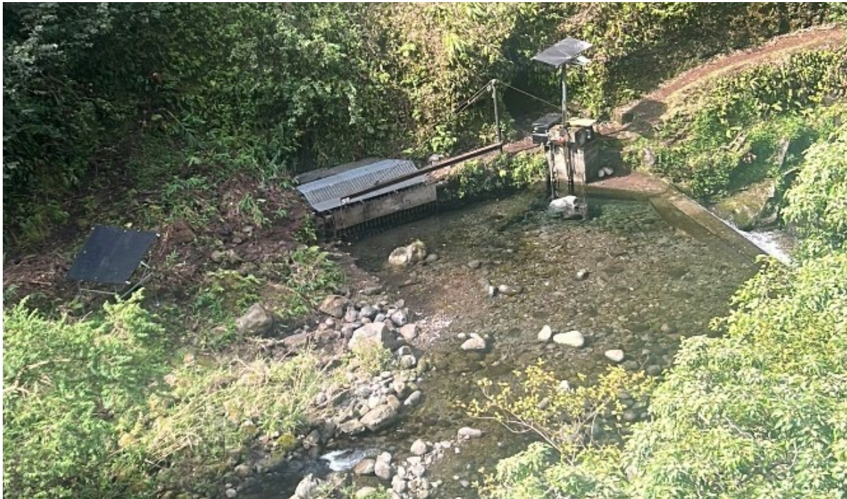
Figure 6. Aerial view of Diversion 770 with intake located on left bank (taken February 5, 2026).
