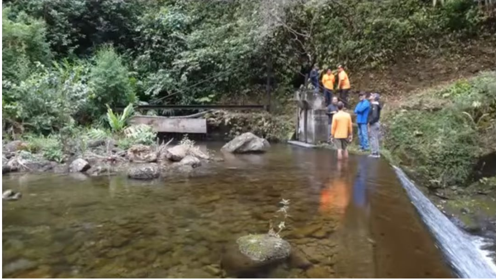
Figure 4: Picture of the dam at Aotaki Weir taken during a site visit in or around May 2025.
