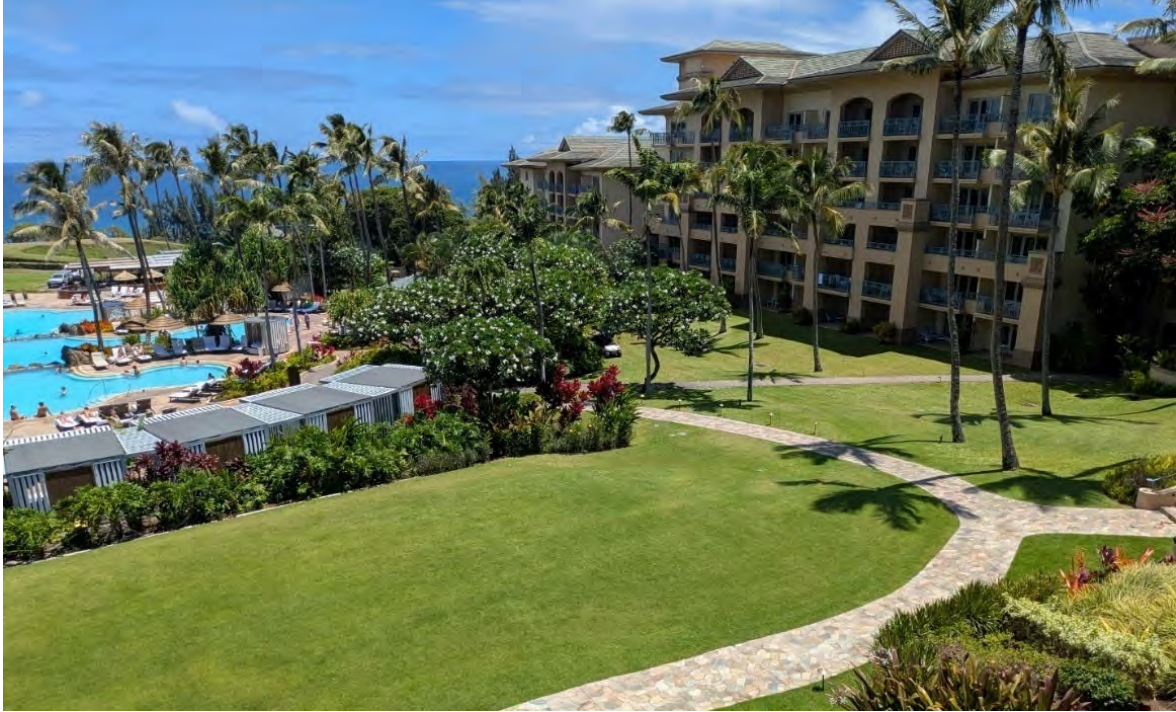
Figure 62: The Ritz-Carlton’s lawns and landscaping appeared to be green and well-watered as recently as August 6, 2025, despite it being subject to the same curtailment orders as other homes and businesses in Kapalua.
