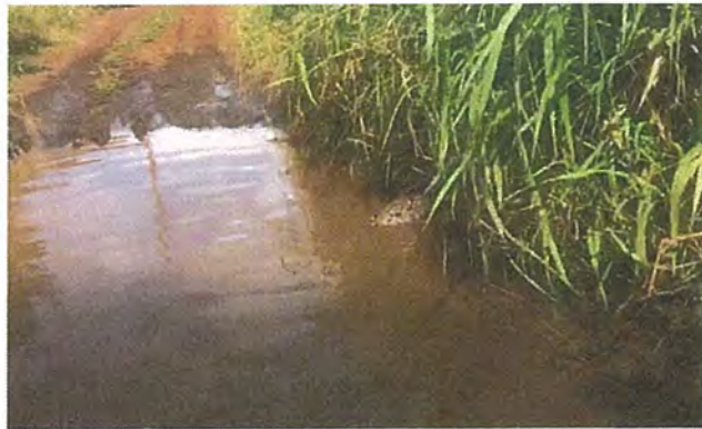
Fig. 4 (right) Water from Wahikuli flume crossing cane haul road. Screenshot of video taken by Wili Wood on Dec. 4, 2018.
