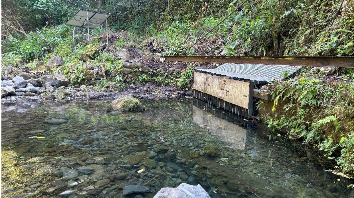
Figure 7. Close up view of trash rack on left bank at Diversion 770 (taken February 5, 2026).
