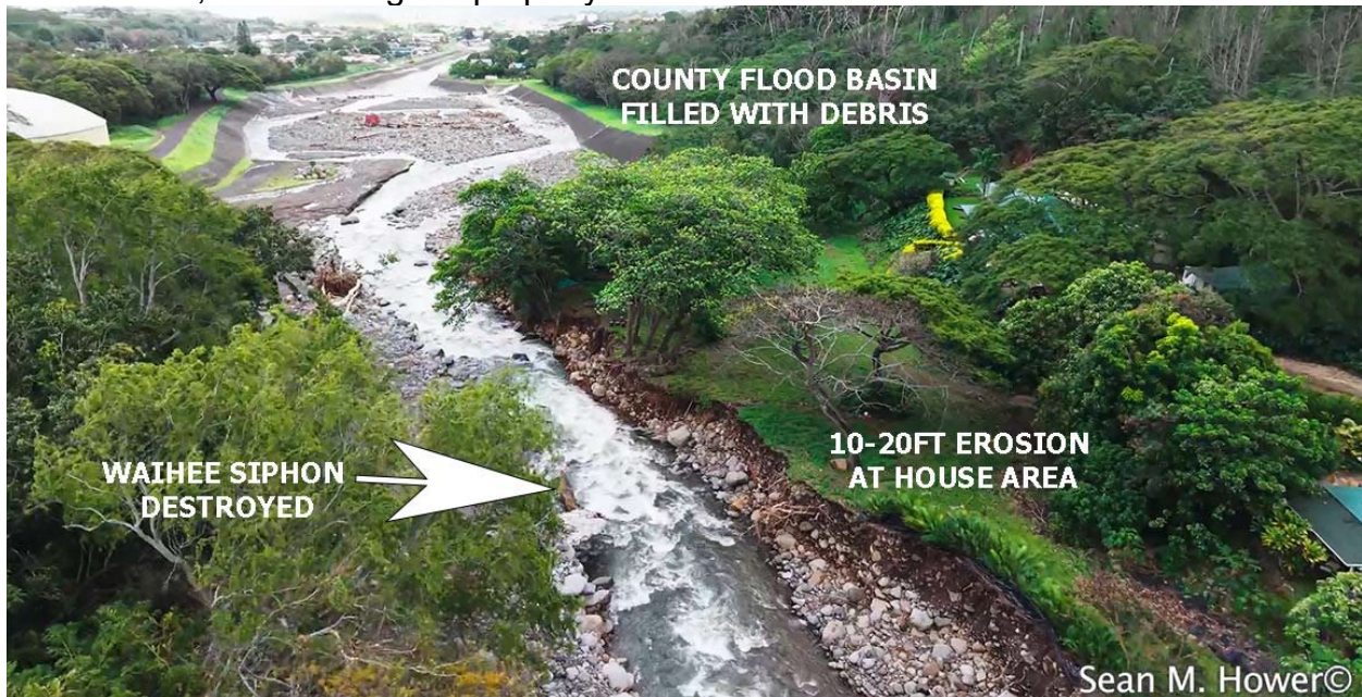
Figure 3. View of Horcajo property damage on right bank of stream, looking downstream, at lower edge of property.
