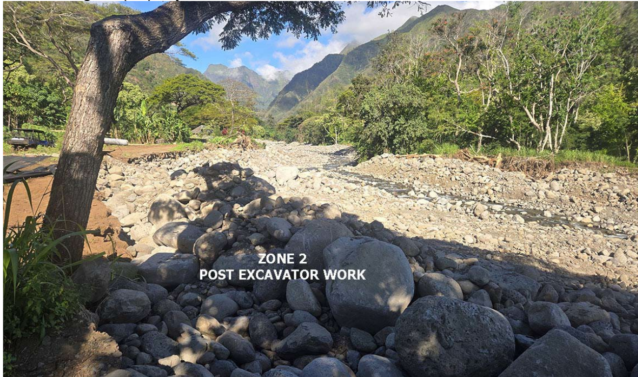
Figure 5. View of Horcajo property damage on right bank of stream, looking upstream, at lower edge of property.
