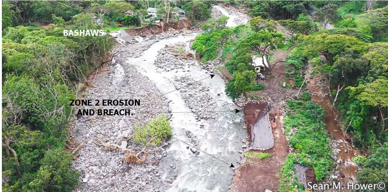
Figure 2. View of Horcajo property damage on right bank of stream, looking downstream, from upper edge of property.
