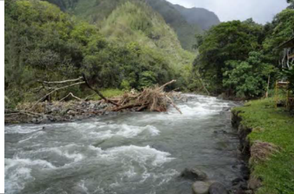
Image 3. Excavator work finished. Bottom of image showing rock berm that was made to protect property and structure. Off in the distance parallel to mountain side, rock berm made to reroute river way from property and structures. This is where the county rerouted the river after the 2016 flood.
