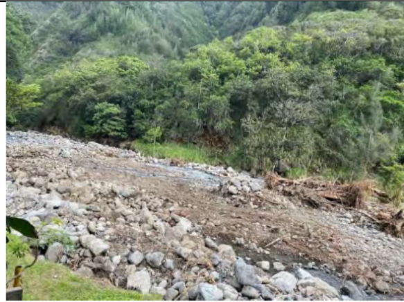
Image 3. Excavator work finished. Bottom of image showing rock berm that was made to protect property and structure. Off in the distance parallel to mountain side, rock berm made to reroute river way from property and structures. This is where the county rerouted the river after the 2016 flood.
