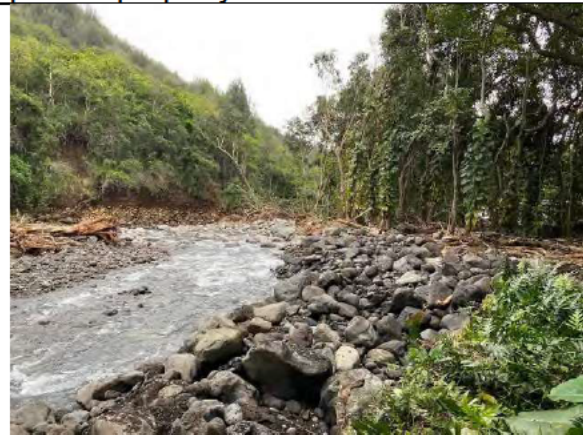
Image 12. Excavator work done. Continuation from Image 10 and 11 looking down river. Far right of image show rock berm that was made to help protect property.
