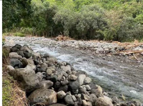
Image 12. Excavator work done. Continuation from Image 10 and 11 looking down river. Far right of image show rock berm that was made to help protect property.
