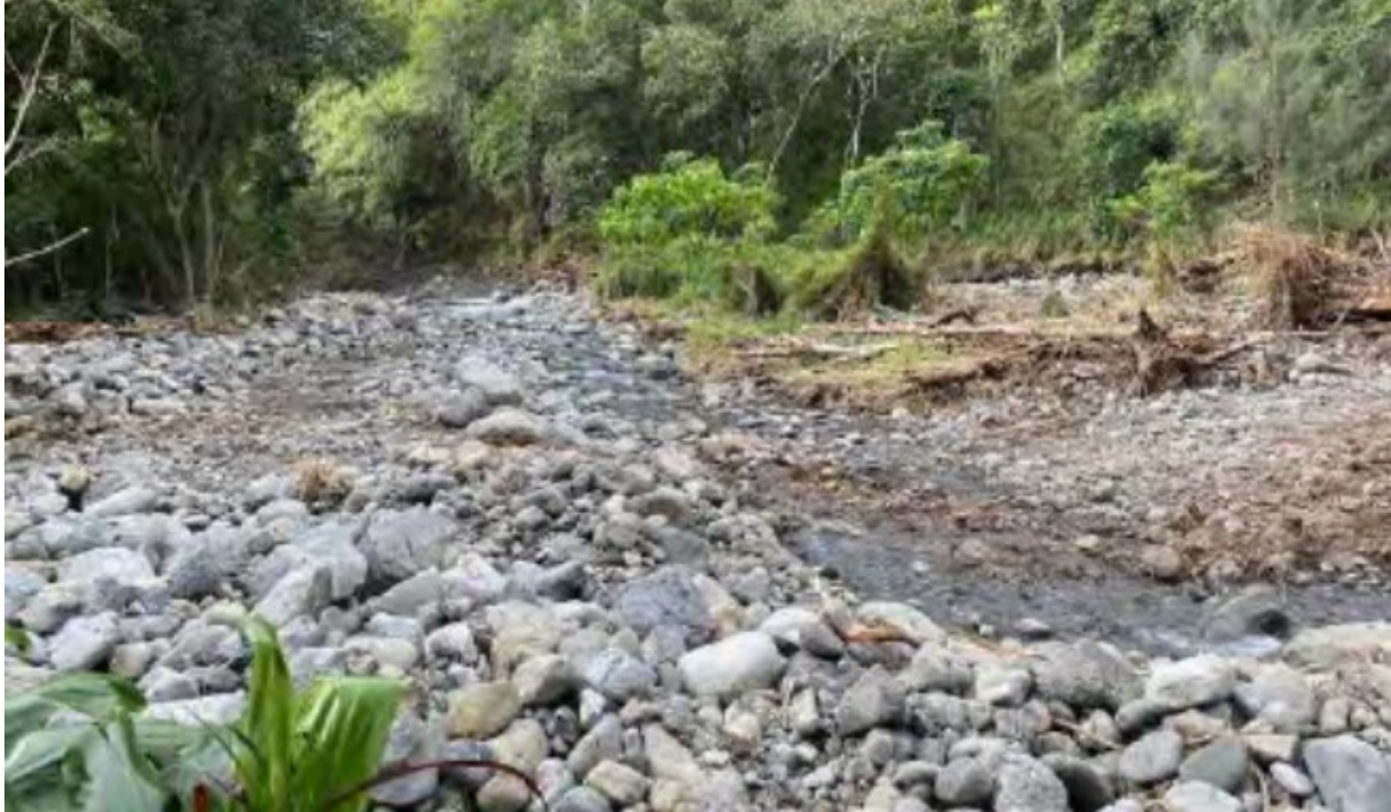
Figure 5. View from right bank of river, looking upstream, with rock berm created in the foreground at edge of property to divert streamflow toward the opposite left bank.
