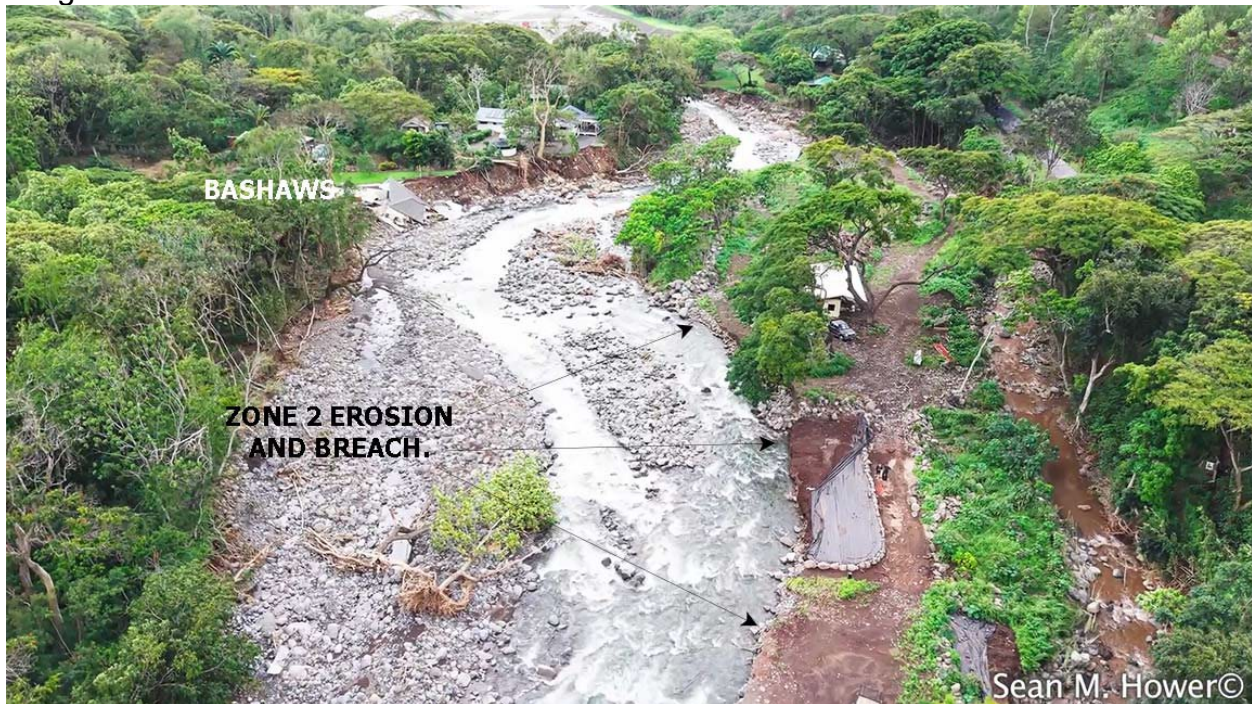
Figure 2. View of property damage on Wailuku River. Image by Robert Horcajo. Juergensmeyer property is located on the left bank of the river in the lower left of the image.
